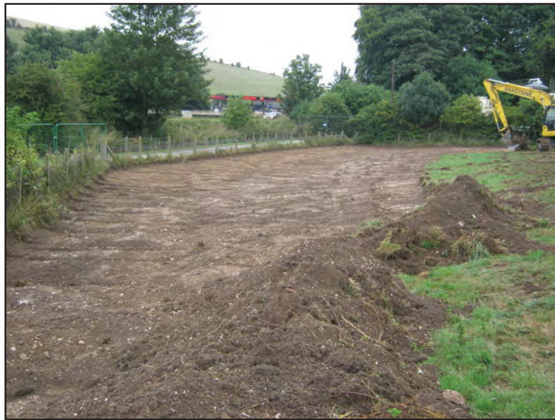
Topsoil stripping of excavation area, facing northeast
