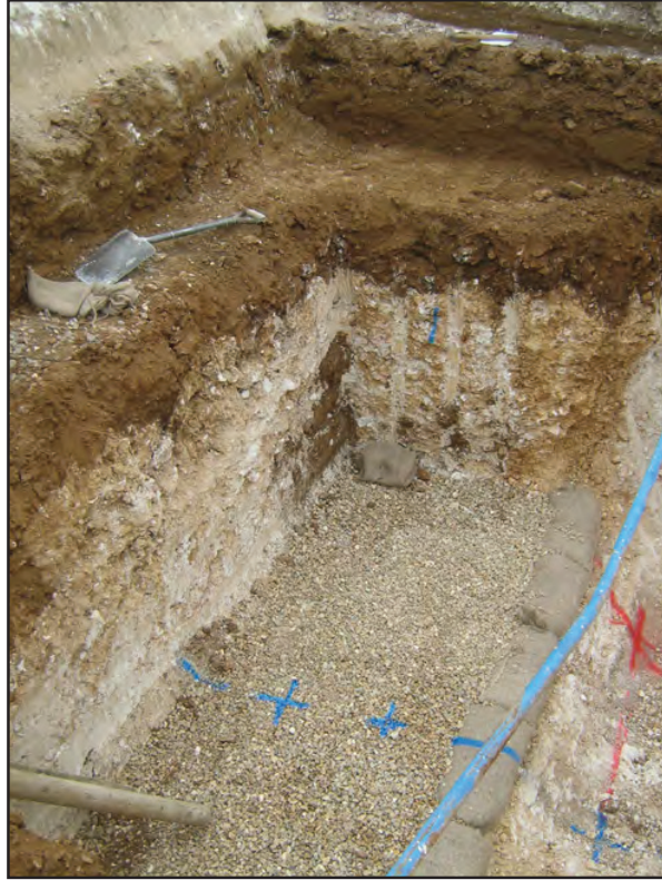
Pipe trench excavation, facing northeast.
