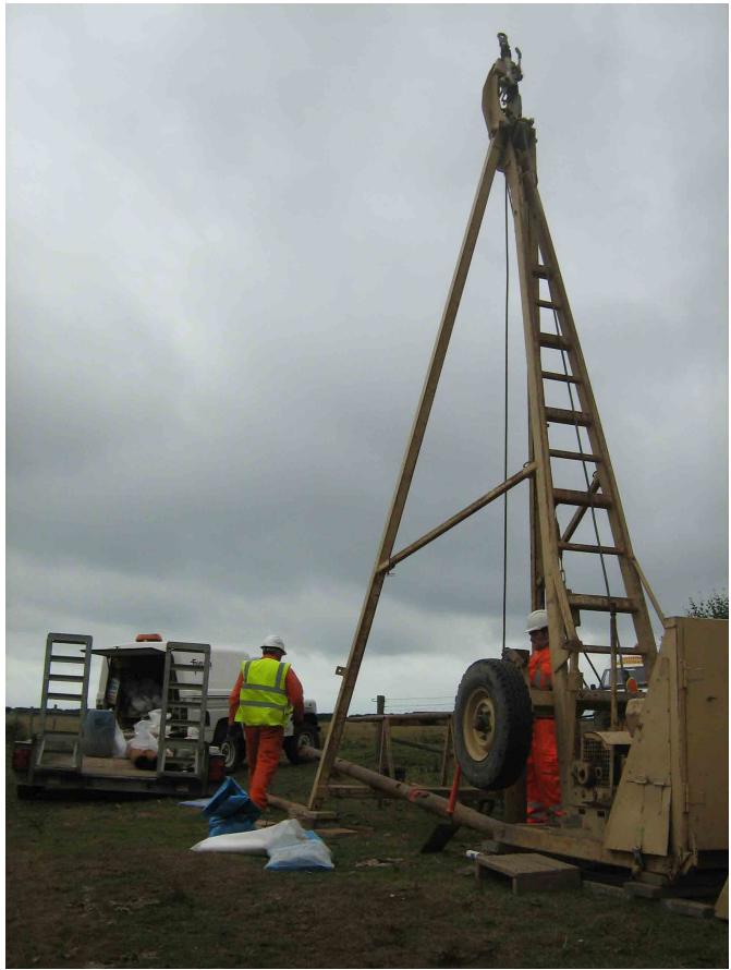
Fig. 3.1: Cable percussion bore hole
