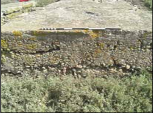
Fig. 4.3: Structure B detail, showing fine grained concrete render
