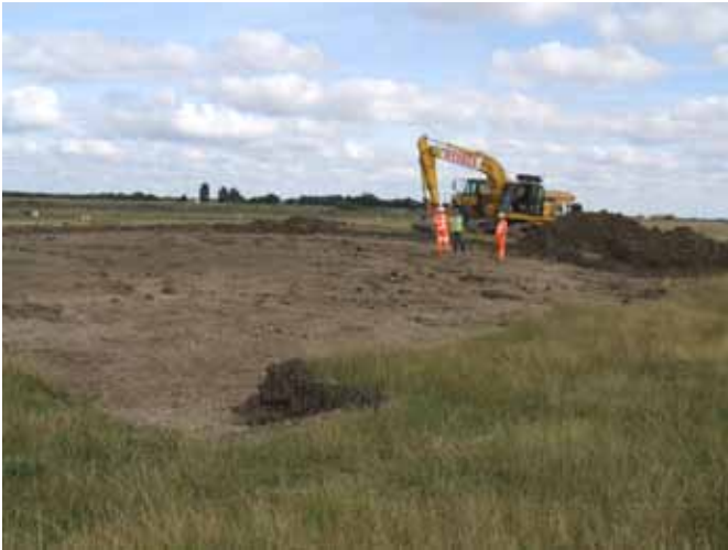
Fig 3.2: Topsoil strip over shingle ridges in field 6
