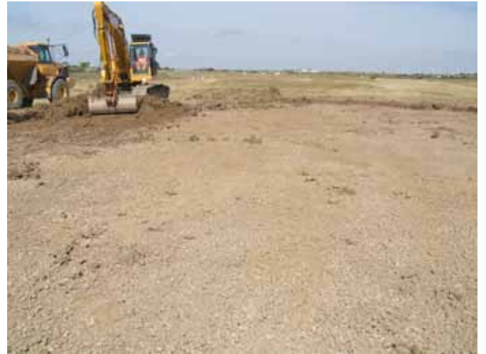
Fig 3.3: Topsoil strip over shingle ridges in field 6
