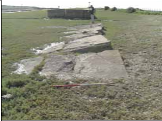
Fig. 4.1: Structure B, looking south-east
