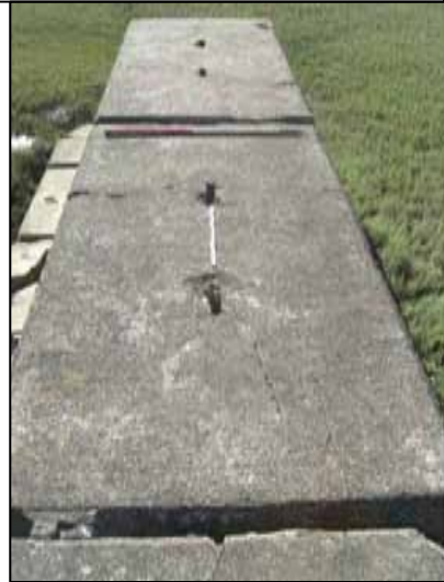
Fig. 3.3: Cast slots and chamfered edges
