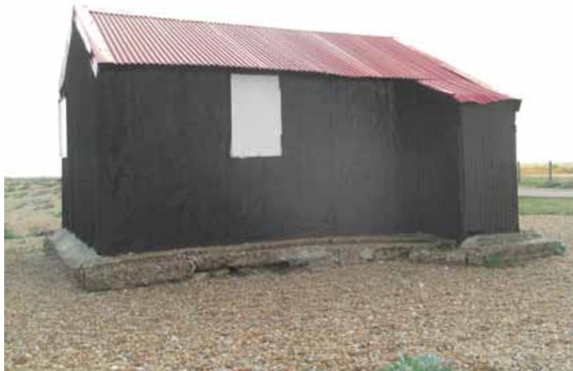
Fig. 8.2 Concrete base to fishing hut at the mouth of the Rother
