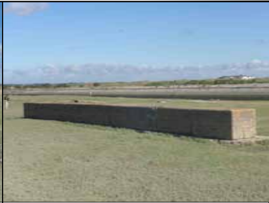
Fig. 3.2: Structure A, looking north
