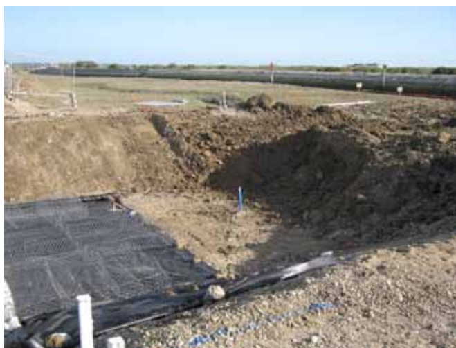
Fig 3.3: Excavation of channel to River Rother
