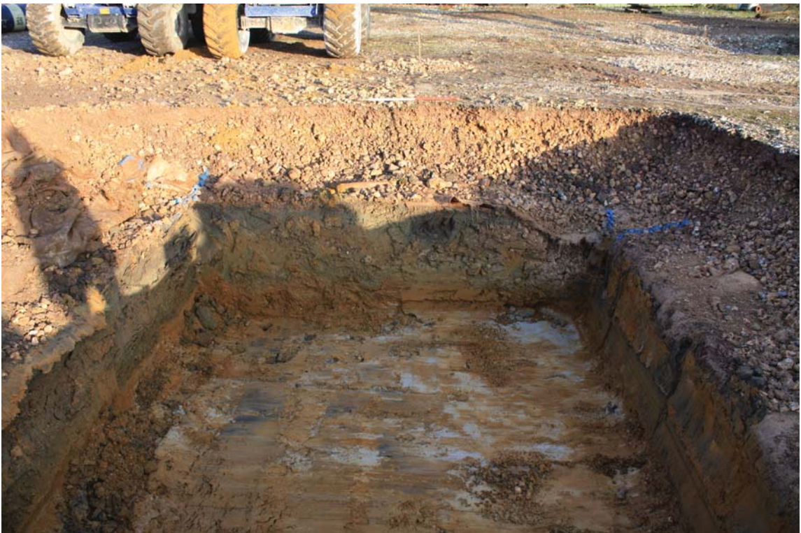
Fig. 3.2: Section through groundworks at limit of observations (within marine sand)
