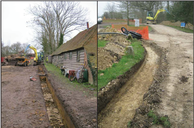
Fig. 2.1: Pipe trench looking north-east
