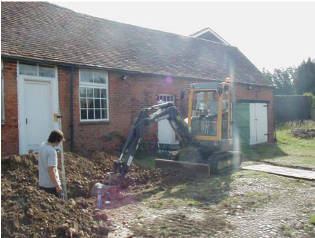
DP 1 Excavation of drainage trench. View south-east
