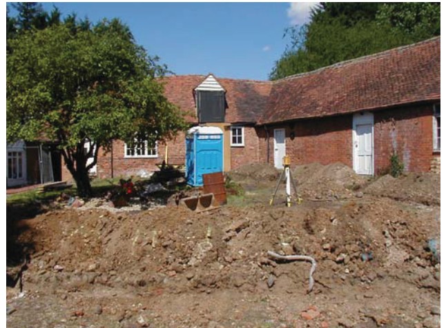
DP 2 General view of area of excavation. View north
