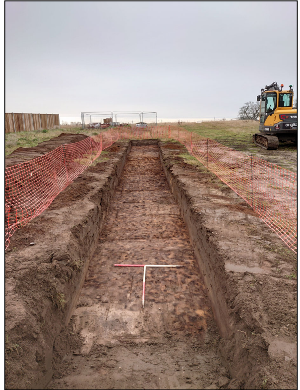
2 Trench 1 looking east
