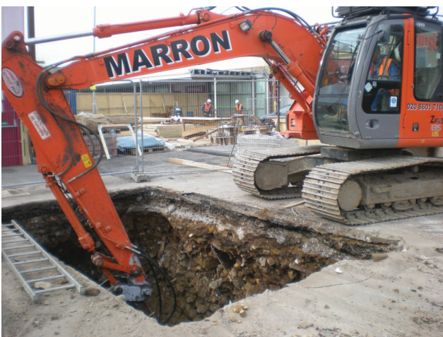
DP 5. Excavation of Trench 5. View W.
