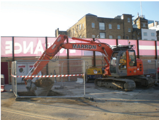
DP 3. Excavation of Trench 1. View SE.
