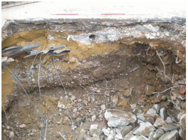
DP 24. Trench 6, section SW. View SW.
