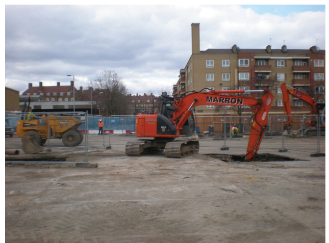
DP 6. Excavation of Trench 6. View NW.
