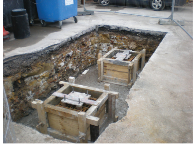
DP 20. Trench 4 with foundation pad. View S.
