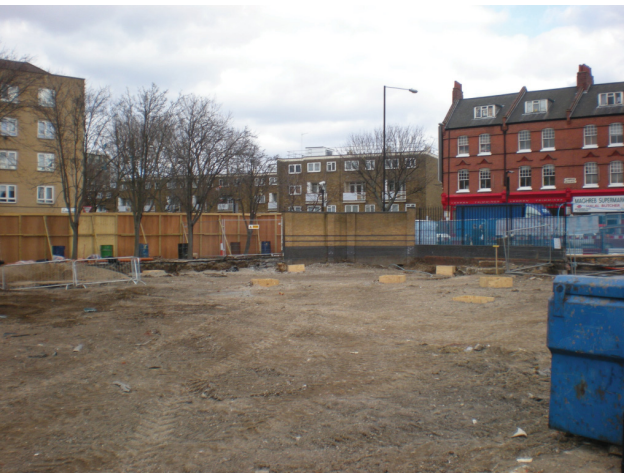
DP 9. E part of the site. View NNE.
