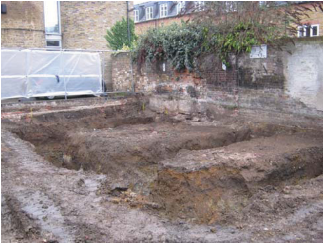
DP 3. Foundation trenches. View W.
