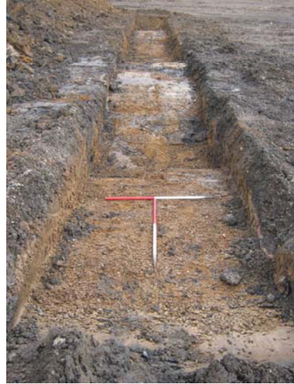
DP 20. Trench 5. View NNW.
