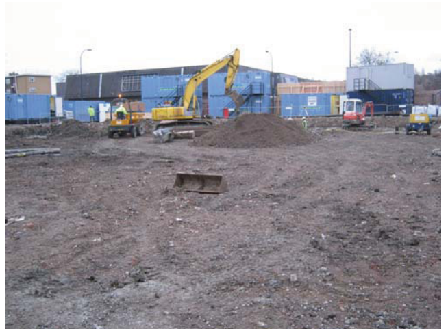
DP 2. Central part of the site before excavation. View N.
