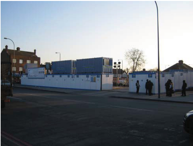
DP 1. The site. View S from Bromley Road.
