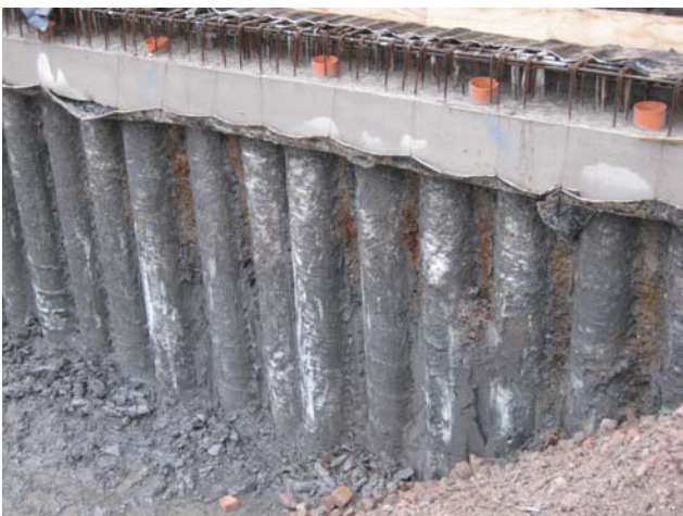
DP 5. SW side of the site. Sample section 1. View SSE.
