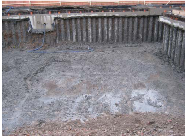
DP 4. S part of the site. View SE.
