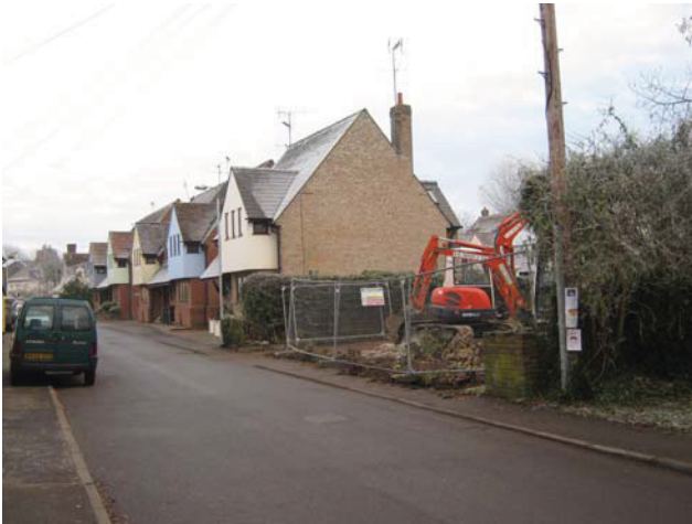
DP 1. South Street, Great Chesterford, Essex. View ESE.
