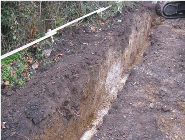
DP 3. E foundation trench. View SSE.
