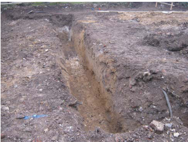
DP 5. S foundation trench. View WNW.
