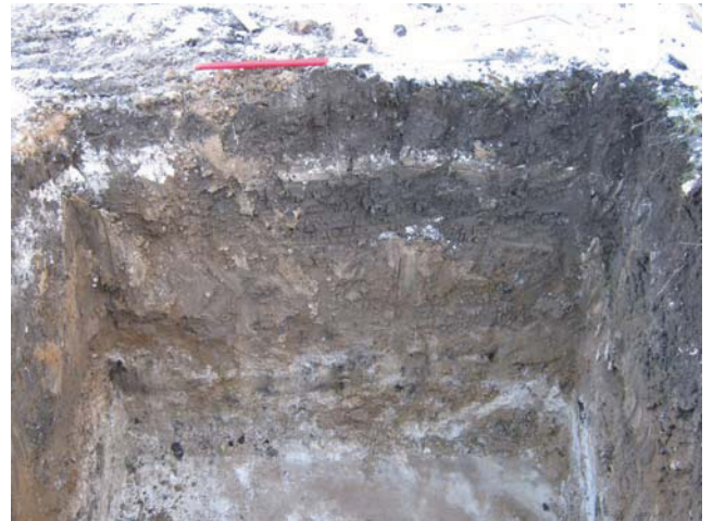
DP 10. Trench for a new soakway. Sample section 3. View E.
