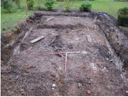
General site shot, garage footings, looking south-west.
