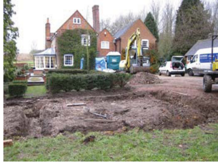
General site shot, garage footings with house in background.
