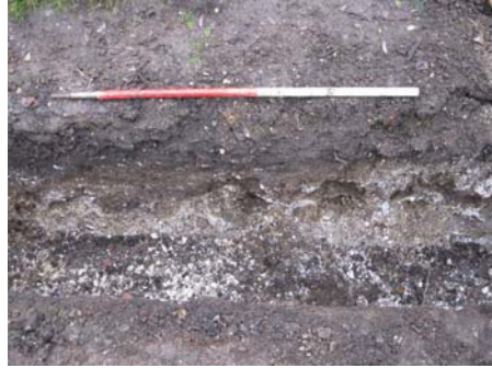
Post-excavation shot of footings, Sample Section 2, looking south-west.
