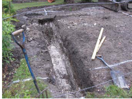
Excavated garage footings, facing south-west.
