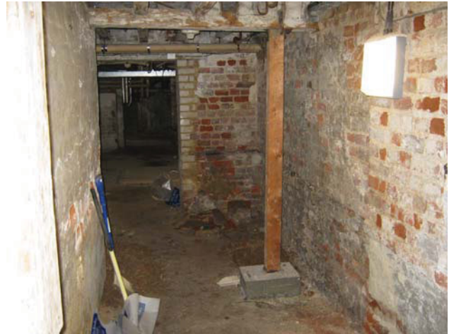
DP 4. Basement with Trial Pit 2. View N.
