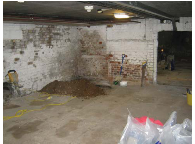
DP 2. Basement of the house with Trial Pit 1. View SW.
