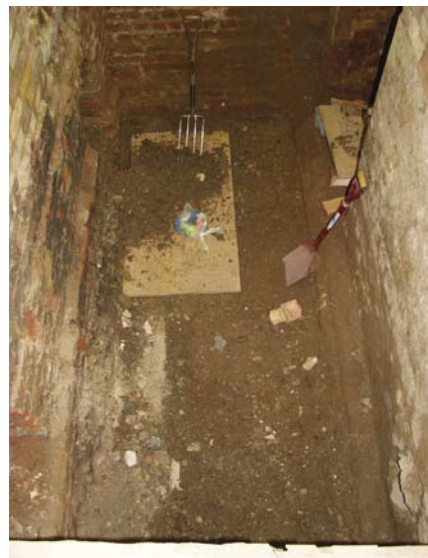
DP 6. Lift Pit. View W.
