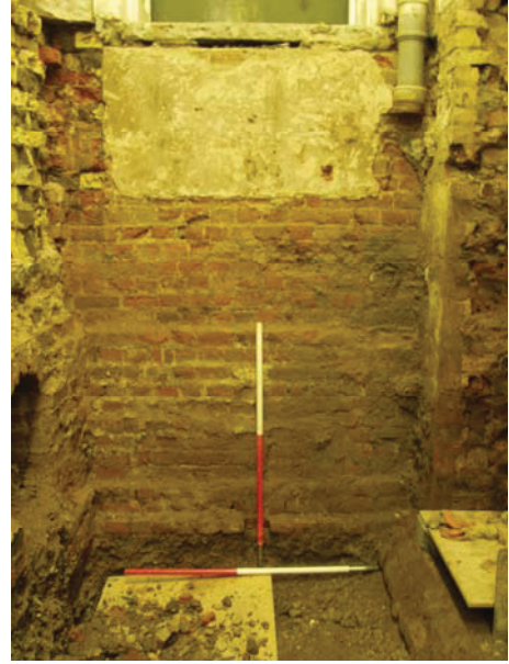
DP 8. Lift Pit. E wall, view W.
