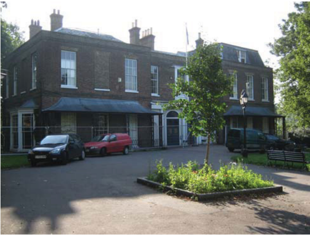
DP 1. Millfield house, Silver Street, Enfield. View SE.
