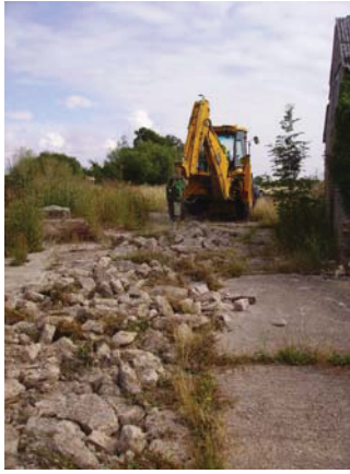
DP1. Breaking concrete. Trench 5
