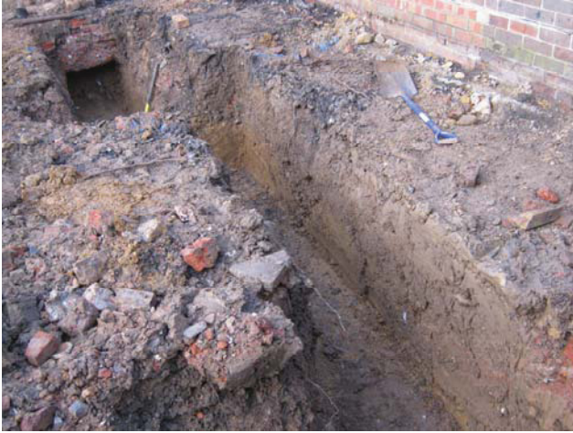
DP 7. N foundation trench. View WNW.
