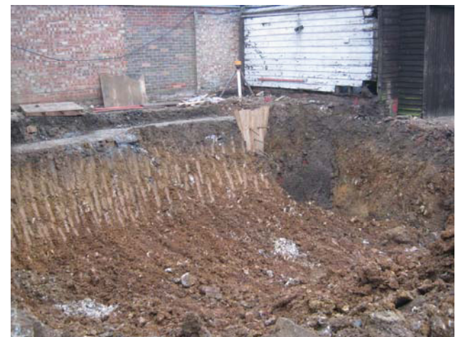
DP 10. Excavation for a new basement. View N.
