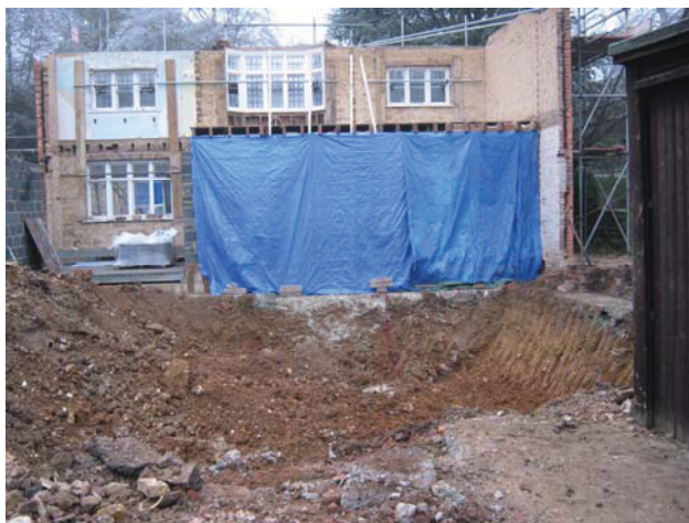
DP 9. Excavation for a new basement. View SW.
