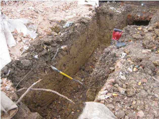
DP 3. SW foundation trench. View NW.
