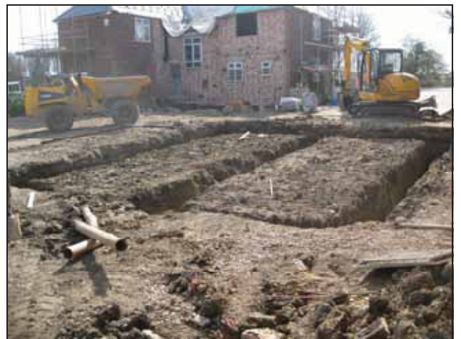
6 Area 3 – Garage footings. Looking south.
