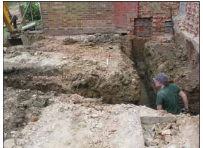
4 Area 2 – Rear Extension. Looking south-east.
