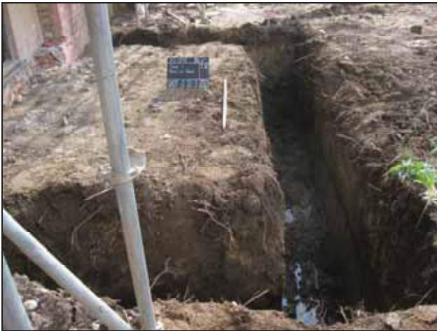
3 Area 1 – Front Extension. Looking south-east.
