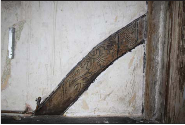
Downward brace on the west wall of Room FF02 showing original painted scheme, taken from the west
