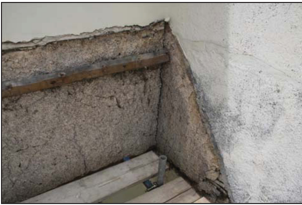
85 Detail of original wattle-and-daub on the south wall (south range), taken from the south
