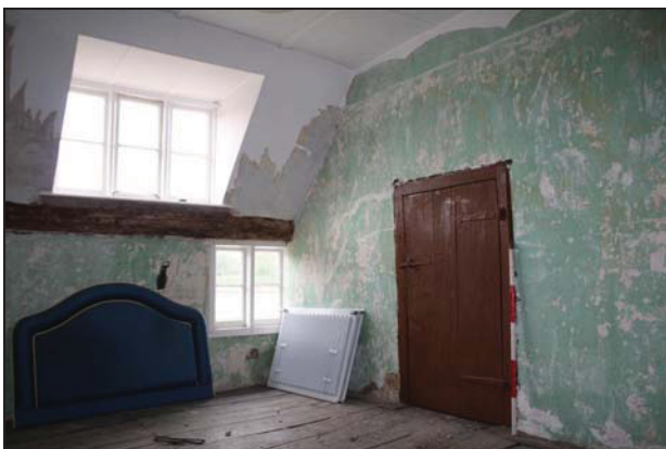
65 South wall of Room FF04, taken from the north-west
