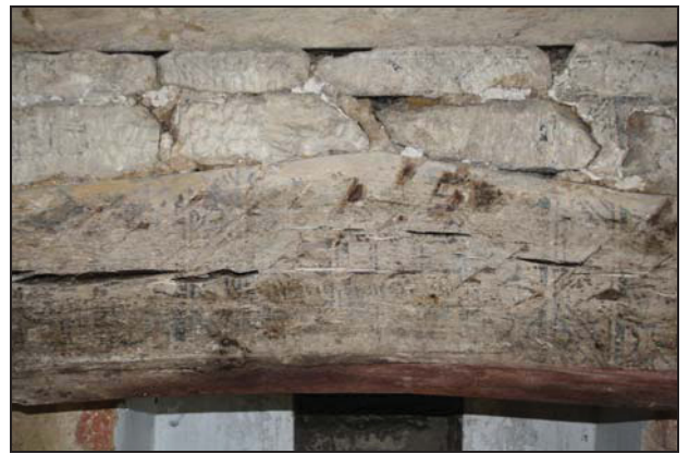
Detail of fire-place lintel in Room FF01 showing original decorative paint scheme, taken from the south
