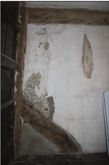
57 Detail of east wall in Room FF01 showing original decorative paint scheme, taken from the west
