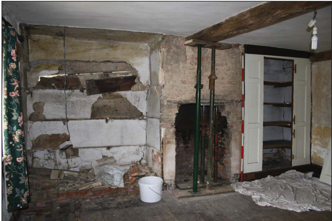
Plate 5 South side of Room GF02, taken from the north (14)
