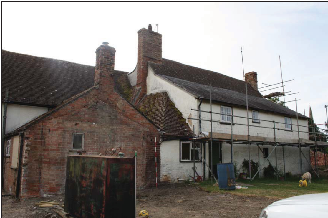
Plate 2 West façade of the assessment building, taken from the north-west (1)
