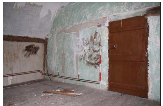
66 North wall of Room FF04, taken from the south-east
