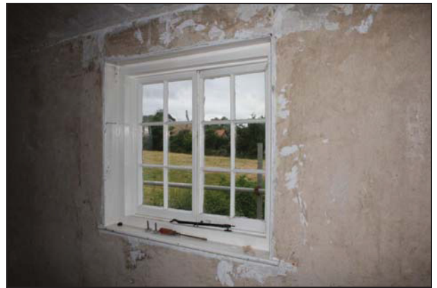
Yorkshire sash window on the east wall of Room FF02, taken from the south-west
