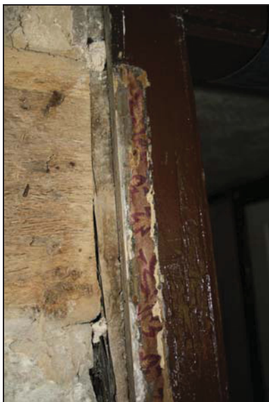
95 Fragment of possible early 19 th century wallpaper adjoining the door jamb of the north door in Room GF01, taken from the south
