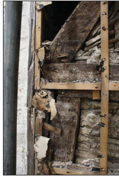
86 Detail of the timber-framing at the west corner of the south gable (south range), taken from the south
