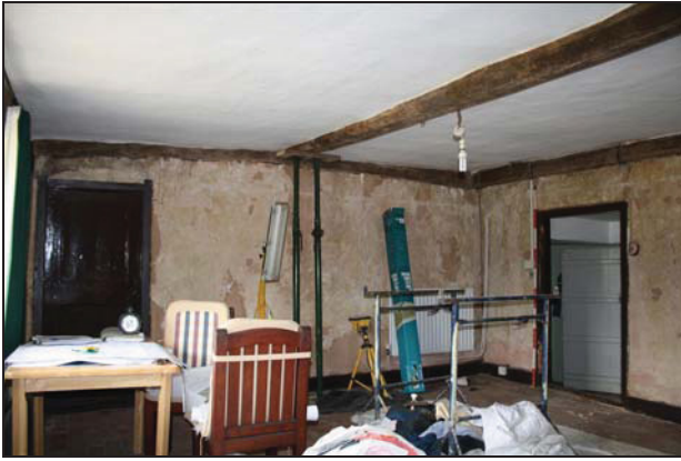
25 West side of Room GF01, taken from the north-east
