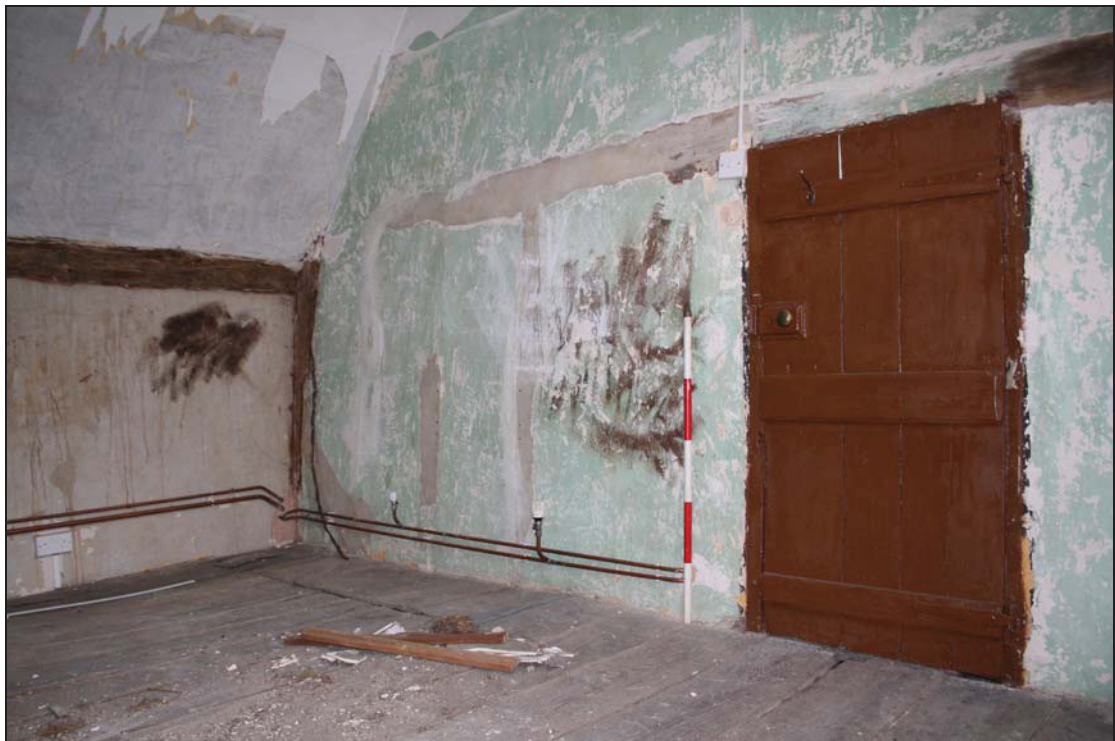
Plate 10 North wall of Room FF04, taken from the south-east (66)
