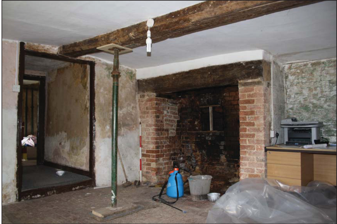
Plate 7 South-west corner of Room GF04 showing fireplace, taken from the north-east (26)
