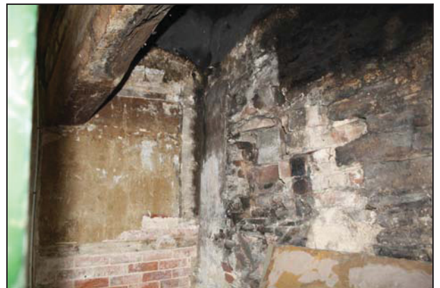
West side of the inglenook showing disturbance for a possible oven along with fine plasterwork, taken from the east
