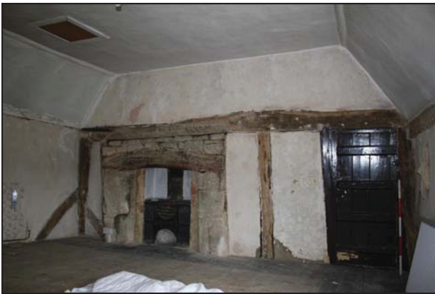
Downward brace on the west wall of Room FF02 showing original painted scheme, taken from the west
