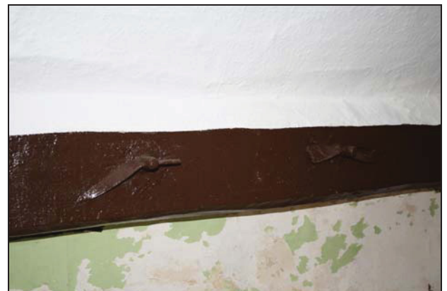
Forelock bolts on the east wall-plate in Room FF05, taken from the north-west
