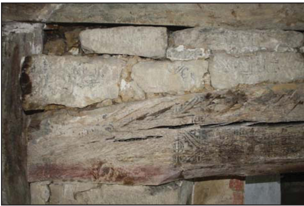
Detail of fire-place lintel in Room FF01 showing original decorative paint scheme, taken from the south
