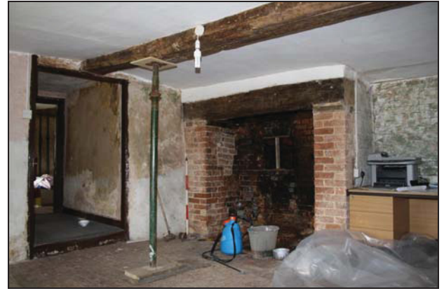
26 South-west corner of Room GF04 showing fireplace, taken from the north-east
