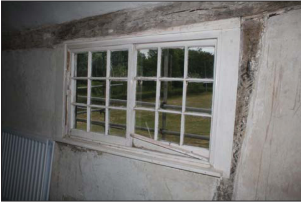
Yorkshire sash window on the east wall of Room FF01, taken from the south-west
