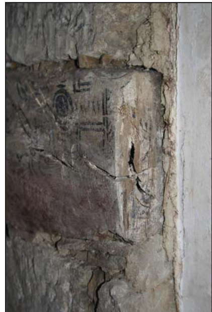
Detail of fire-place lintel in Room FF01 showing original decorative paint scheme, taken from the south
