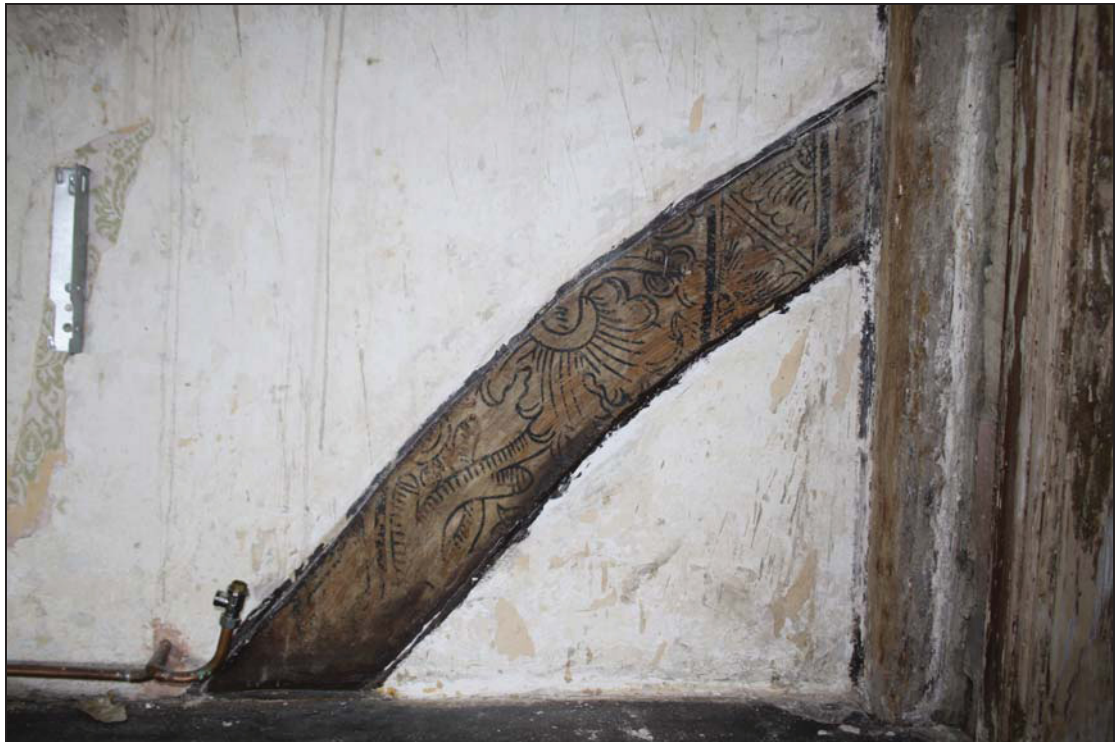
Plate 9 Downward brace on the west wall of Room FF02 showing original painted scheme, taken from the west (43)
