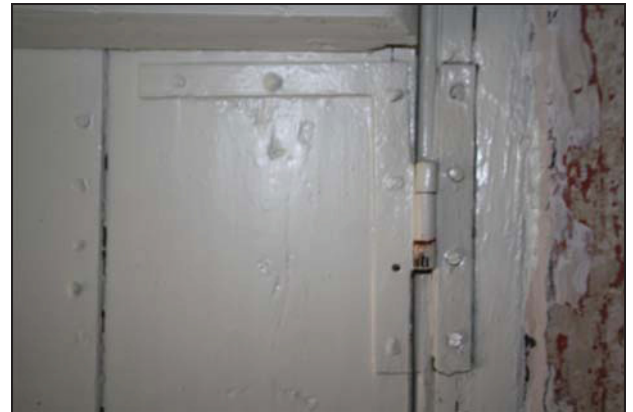
Detail of H-L hinge on the door to Room FF06, taken from the west
