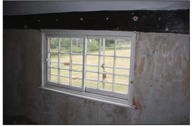
Yorkshire sash window on the east wall of Room FF02, taken from the south-west
