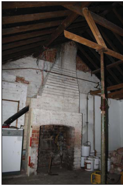
East wall of Room GF09 showing formerly external wall of the main range, taken from the west
