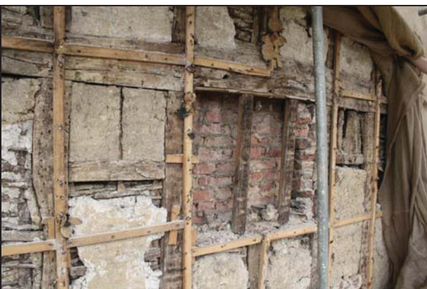
Blocked original tri-partite first-floor window on the south wall (south range), taken from the south-west
