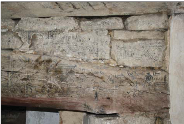
Detail of fire-place lintel in Room FF01 showing original decorative paint scheme, taken from the south
