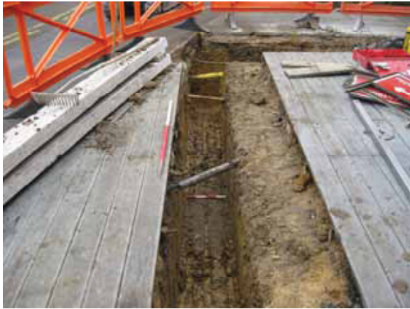
1 Post-excavation view of footings. Looking north-east.
