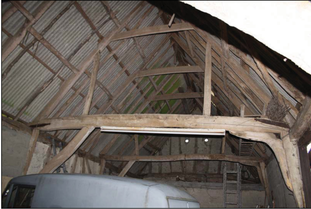
Plate 3 Truss 3, taken from the south-west (DP 24)
