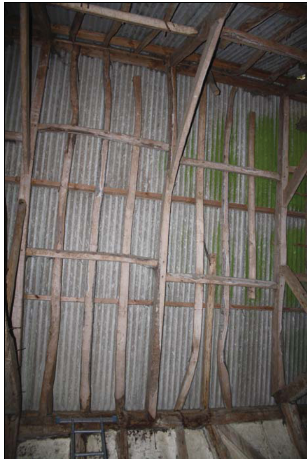
Plate 6 Northern roof panel, Bay 3, taken from the south-west (DP 29)
