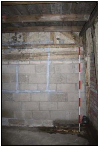
Wattle and daub panels preserved within the outer east wall, taken from the west
