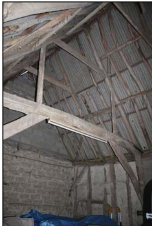
Truss 2 and clay lump wall (Truss 1), taken from the south-east
