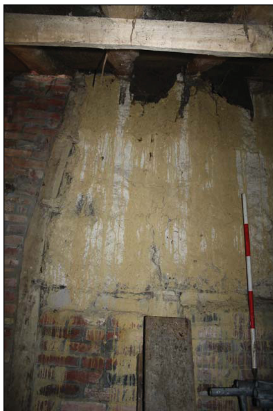
Plate 8 Wattle and daub panels preserved within the external barn wall, taken from the south-east (DP 10)
