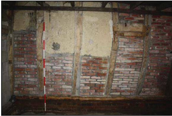
Wattle and daub panels preserved within the outer east wall, taken from the west
