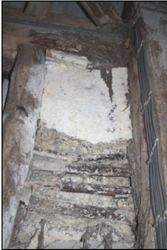
Wattle and daub panel with exposed horizontal laths, Bay 2, taken from the north
