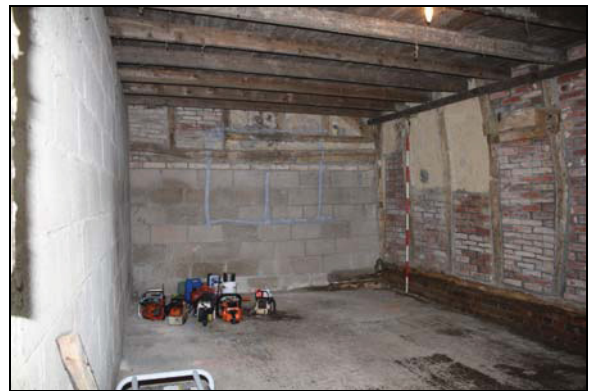
Wattle and daub panels preserved within the external barn wall, taken from the south-east
