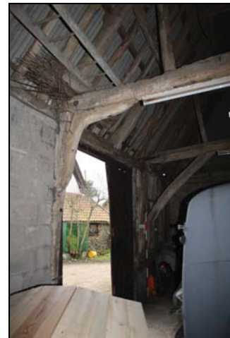
Truss 3 with kneeler brace, taken from the north-east
