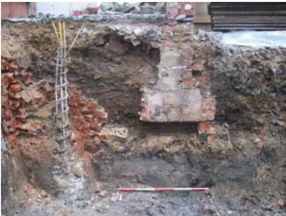
DP 17. Building Plot B (area of 'strip, map and record'), north-east-facing section (Sample Section 5), southern part. View WSW.
