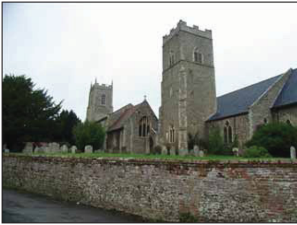
1 St Michael's (background) and St Mary's. Looking north-west.
