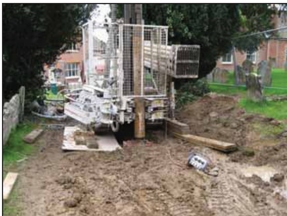
11 Drilling rig over central borehole. Looking south.
