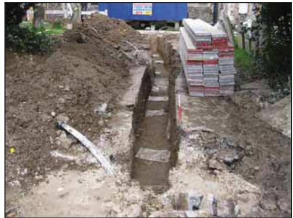
16 North-south trench run, post-excitation. Looking north.
