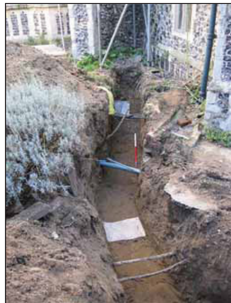
18 North-south trench run beside porch, post-excitation. Looking north.
