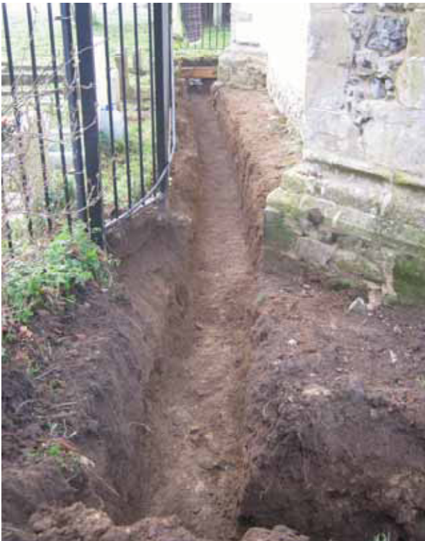
3 Trench for french drain beside east wall of chancel. Looking south.
