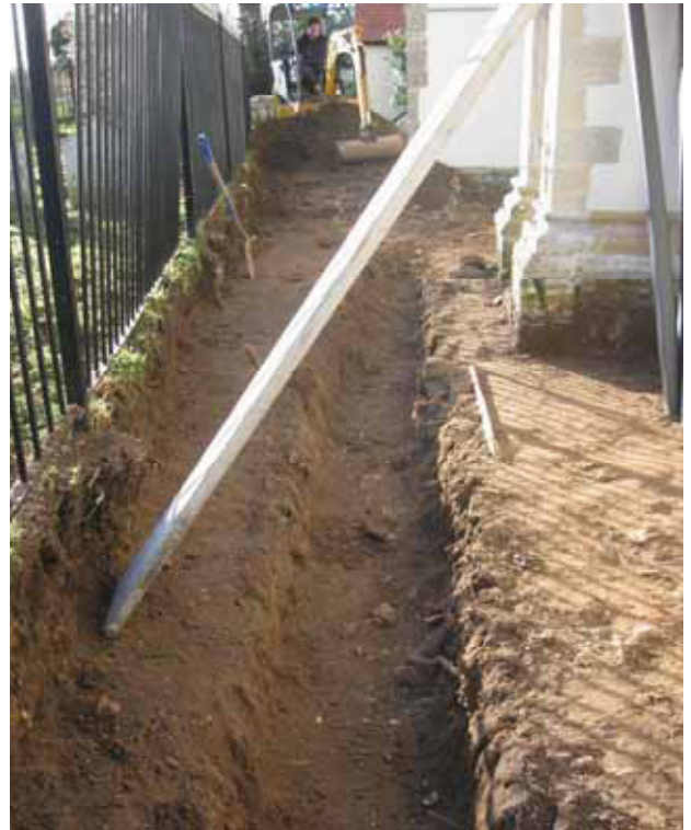
2 Trench for french drain beside south wall of chancel. Looking west.
