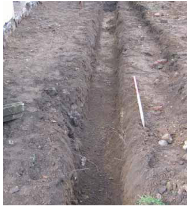
8 Trench for french drain beside north wall of chancel. Looking west.
