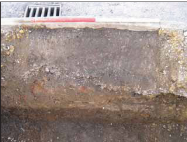
3 Sample Section 2. Looking south.
