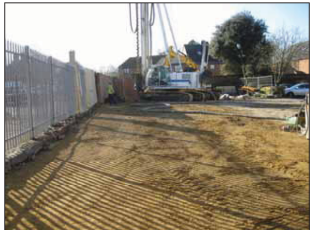
6 General site view & piling rig. Looking south.
