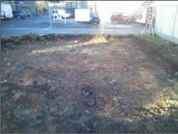
1 General site view. Looking west.
