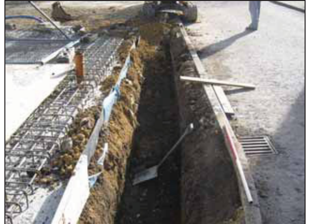
2 Water service trench. Looking east.
