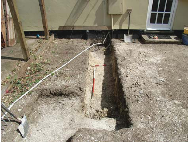
1 Northernmost footing trench. Looking north-east
