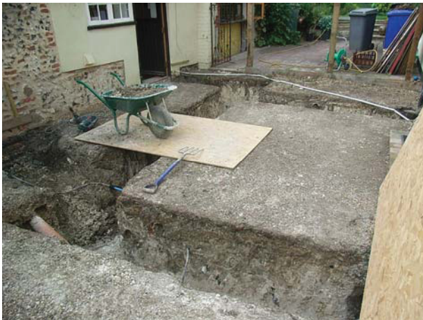
3 General view of southernmost footing trench and connecting trench. Looking north.
