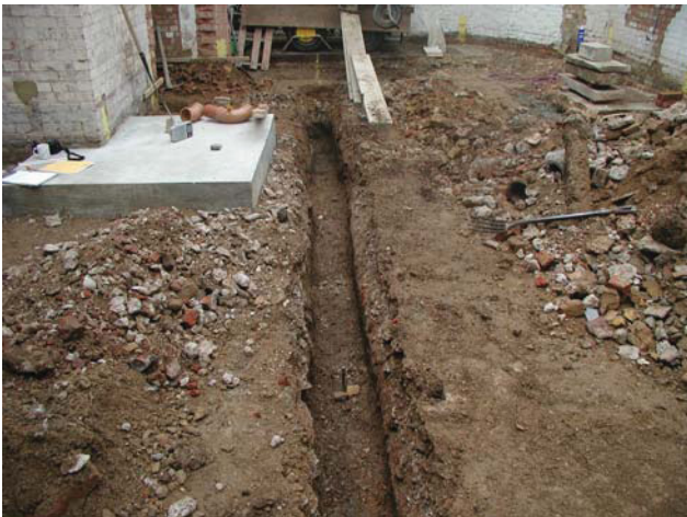
DP 9. S drainage trench. View W.
