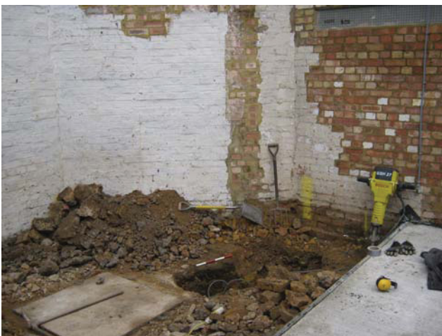
DP 11. NW drainage trench. View NW.
