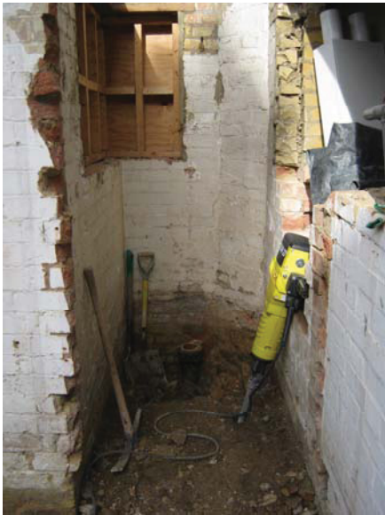
DP 7. Test Pit 3. View W.
