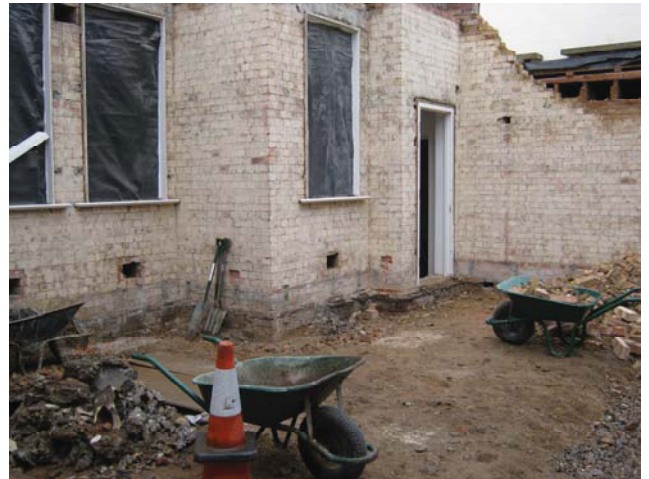
DP 2. SW yard within the building. View SW.
