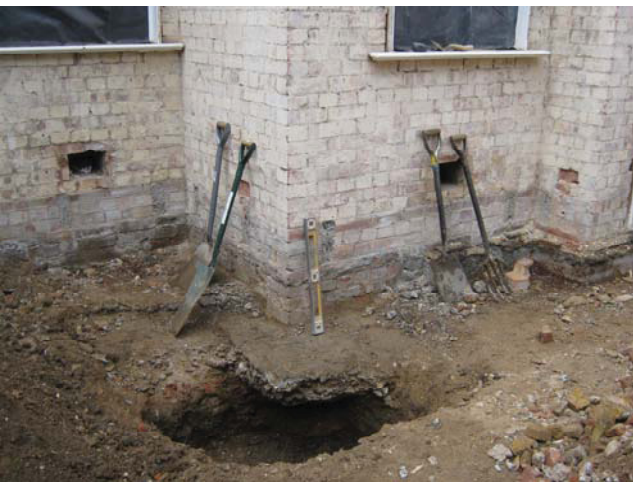
DP 5. Test Pit 2. View SW.
