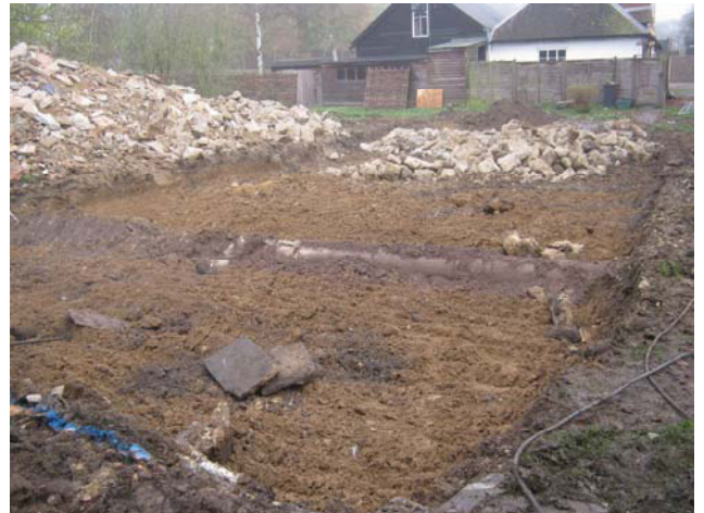
DP 2. The area of ground reduction. View NE.
