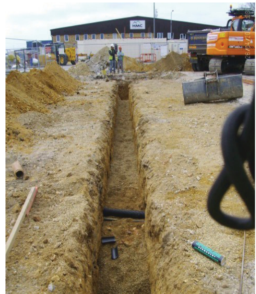
DP16 East/west drainage trench, looking west
