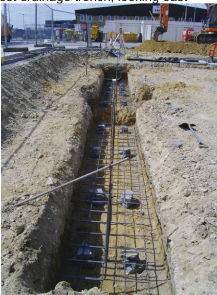
DP17 Extension footings, looking west
