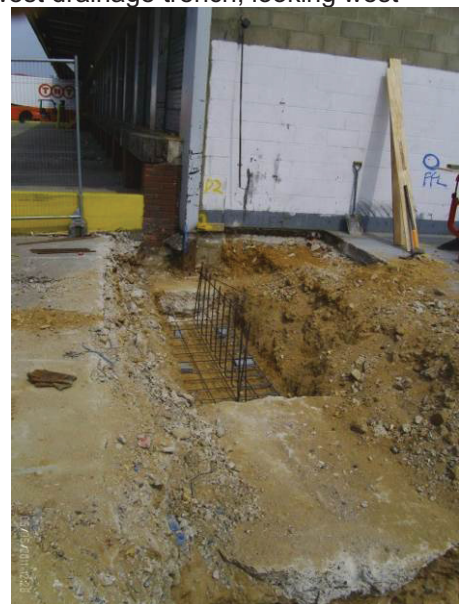
DP18 Extension footings, looking north
