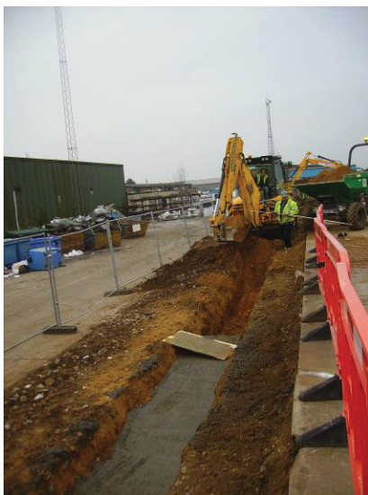
DP11 Excavating wall foundation trench. Looking west.
