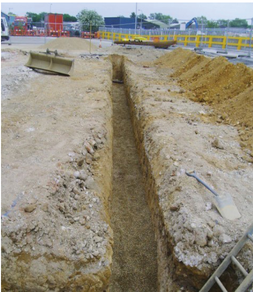
DP15 East/west drainage trench, looking east
