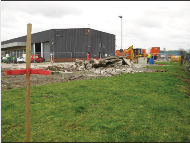
DP1 General view of the site, pre excavation. Looking northeast.
