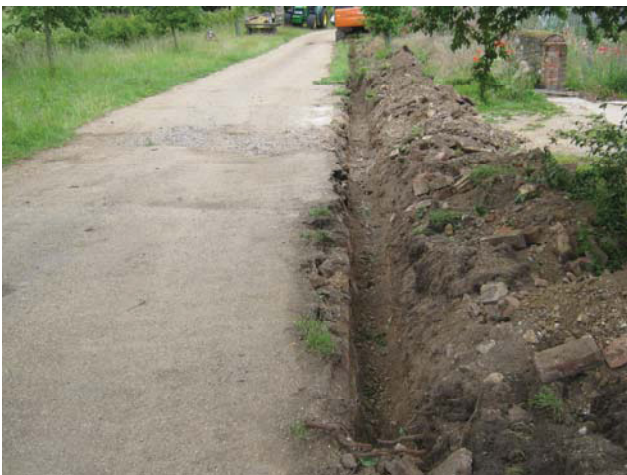
DP 5. Central part of the trench. View SE.
