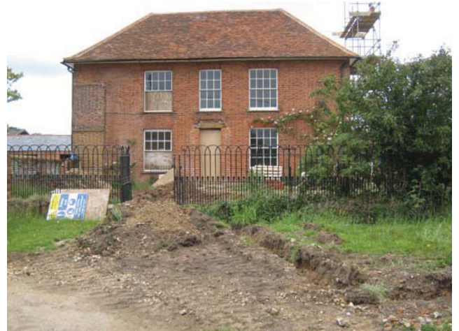
DP 4. Trench extension to the house. View N.
