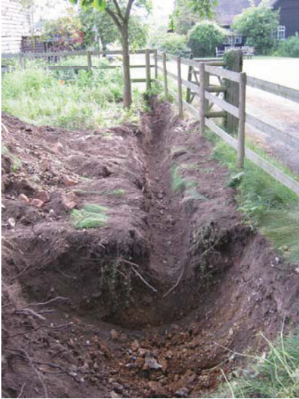
DP 7. S/central part of the trench. View ESE.
