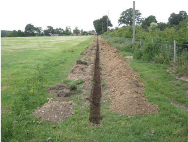
DP 1. Gorhambury estate. NE part of the trench. View SW.
