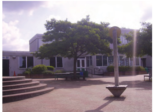
DP 4 Western frontage of the main school building, with an extensive area of hardstanding recreation area and playground
