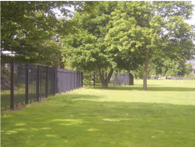
DP 1 Northern boundary of the site demarcated by railings and forming the southern extent of the SAM associated with Barking Abbey
