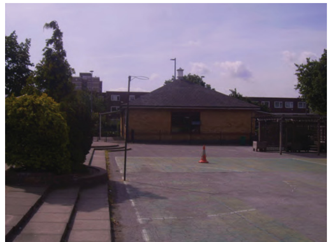
DP 6 Late 20 th century nursery building situated within the central southern section of the site, view south
