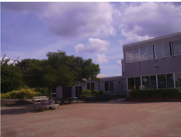
DP 5 Western frontage of the main school building, with further extensive areas of hardstanding recreation area and playground
