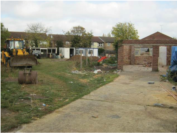
1 General view, looking north-east
