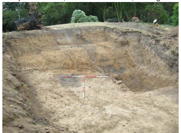
DP 6 Trench after excavation, looking south
