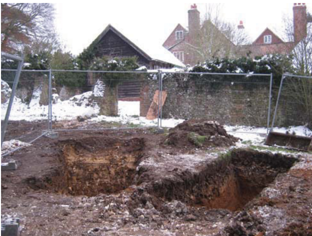
DP 5. Two trenches for a biodigester unit. View NE.
