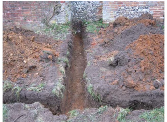
DP 10. Drainage trench to the south of the house. View N.
