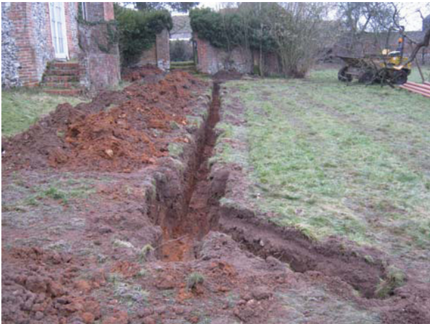
DP 9. Drainage trench to the south of the house. View E.
