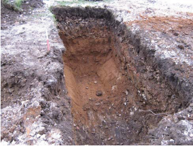
DP 7. S trench for a biodigester unit. View E.
