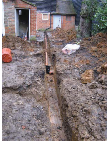
DP 14. Drainage trench to the east of the house. View NNE.
