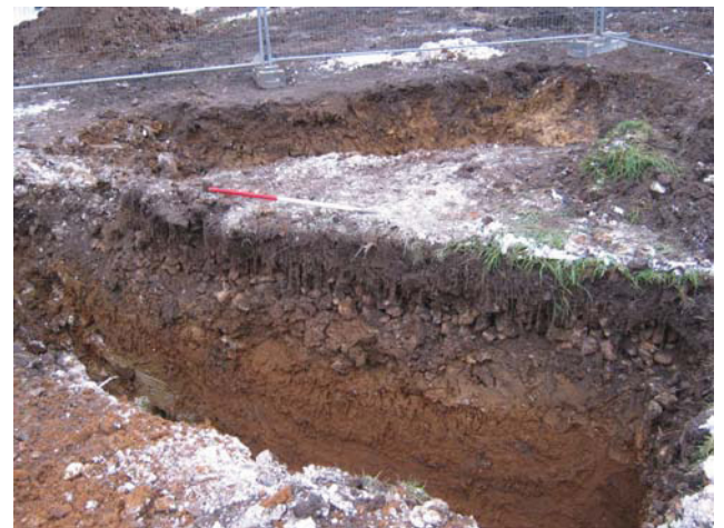
DP 6. S trench for a biodigester unit. View NW.
