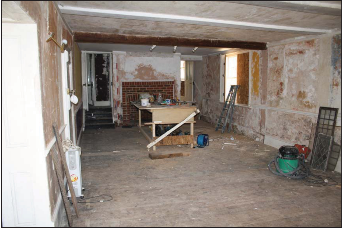
Plate 7 GF01, taken from the south-west (DP 37)
