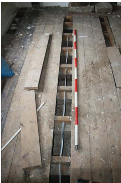
Secondary joisting revealed after removal of floorboards, FF03, taken from the east
