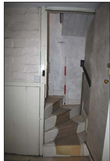
66 Attic stair leading to the second floor, taken from the north
