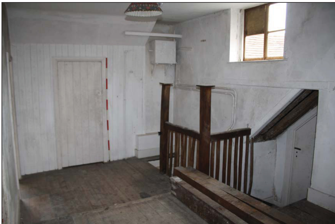
Plate 22 Service range stair vestibule, SF07, taken from the north-west (DP 30)
