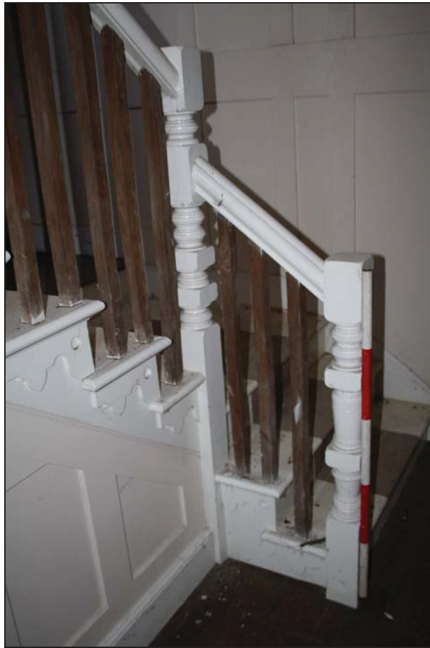
Plate 9 Turned newels and staircase configuration, GF03, taken from the south-west (DP 47)
