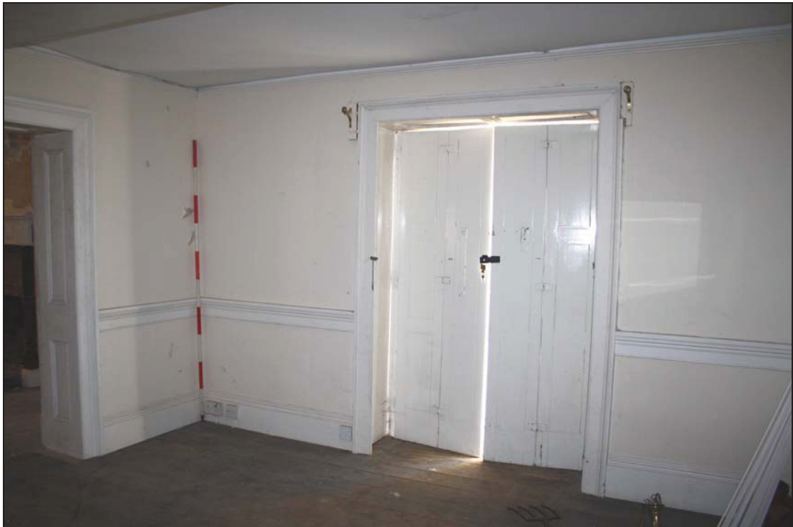
Plate 8 French doors and panelled shutters, GF02, taken from the north-west (DP 43)
