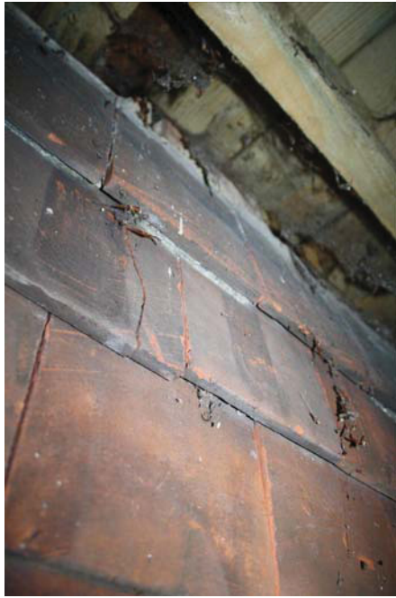
Tiled elevation preserved within the covered valley of the 'M' roof of the historic core, taken from the south
