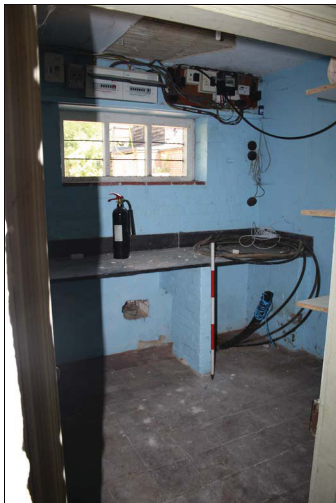
Plate 14 GF08, taken from the south-west (DP 32)
