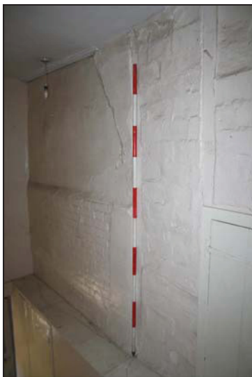
65 Exposed brickwork and rear chimney stack, taken from the north-west
