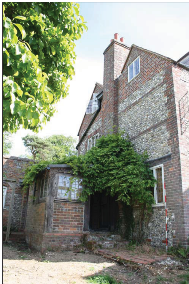
Plate 4 West elevation of the later 20th century extension, taken from the south-west (DP 05)
