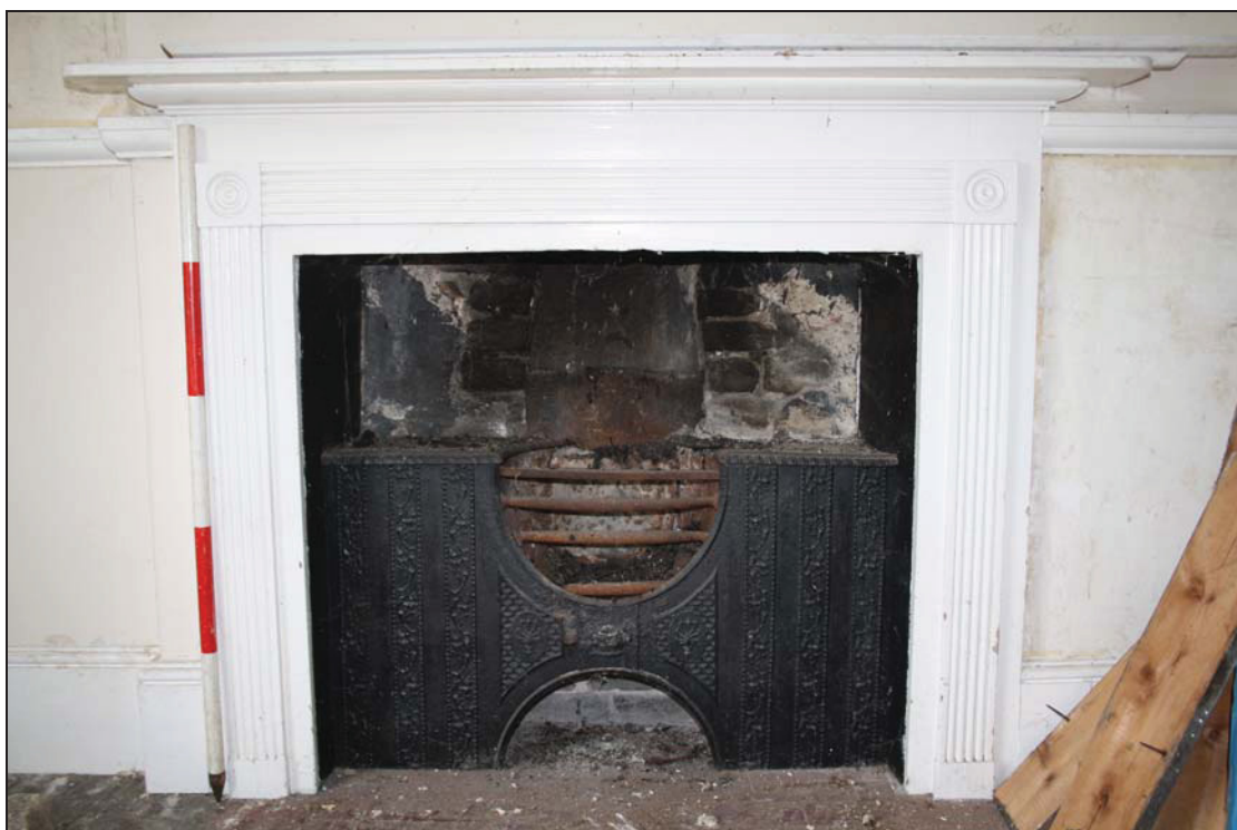
Plate 18 Fireplace with early 19th century surround and hob grate, FF03, taken from the east (DP 105)
