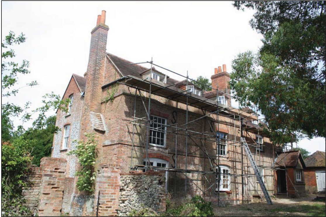
Plate 1 Principal east façade, taken from the south-east (DP 08)
