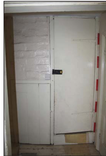
64 Attic stair door and cupboard, first floor, taken from the north
