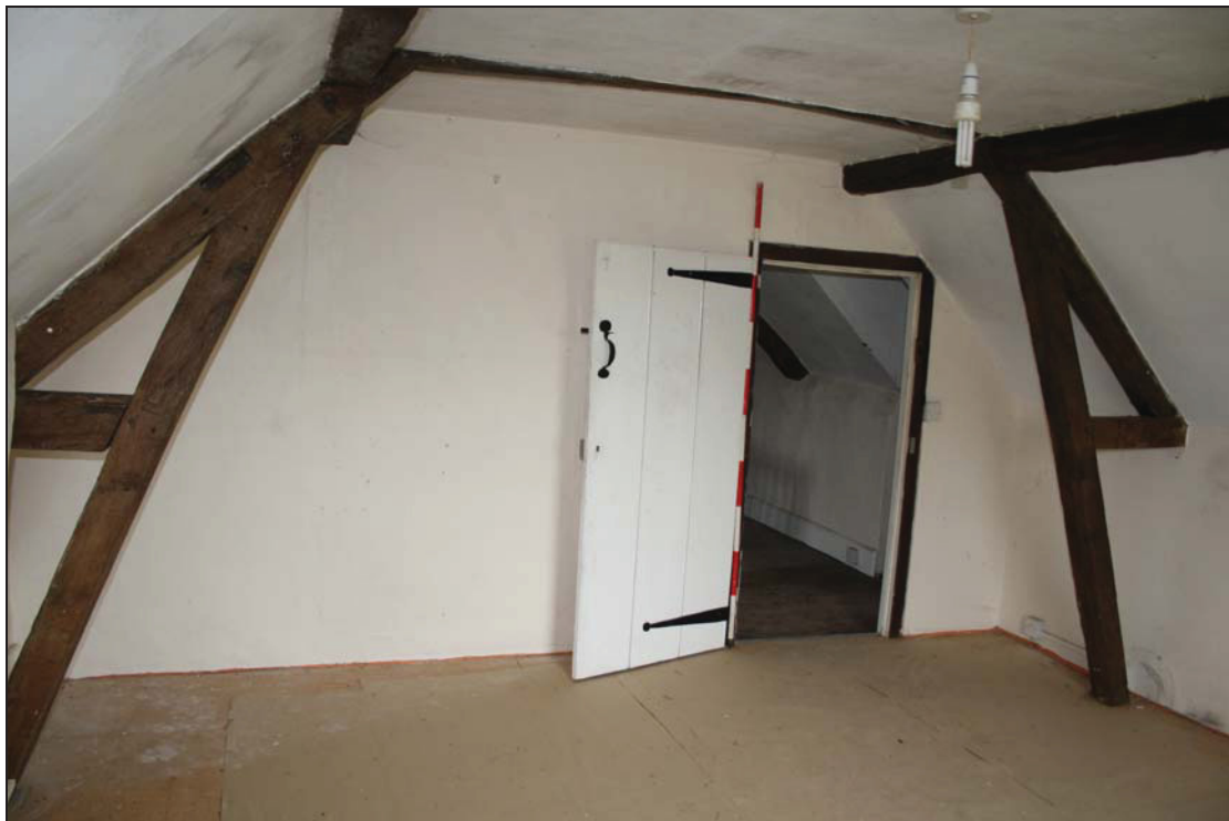
Plate 21 SF03, taken from the north-east (DP 123)
