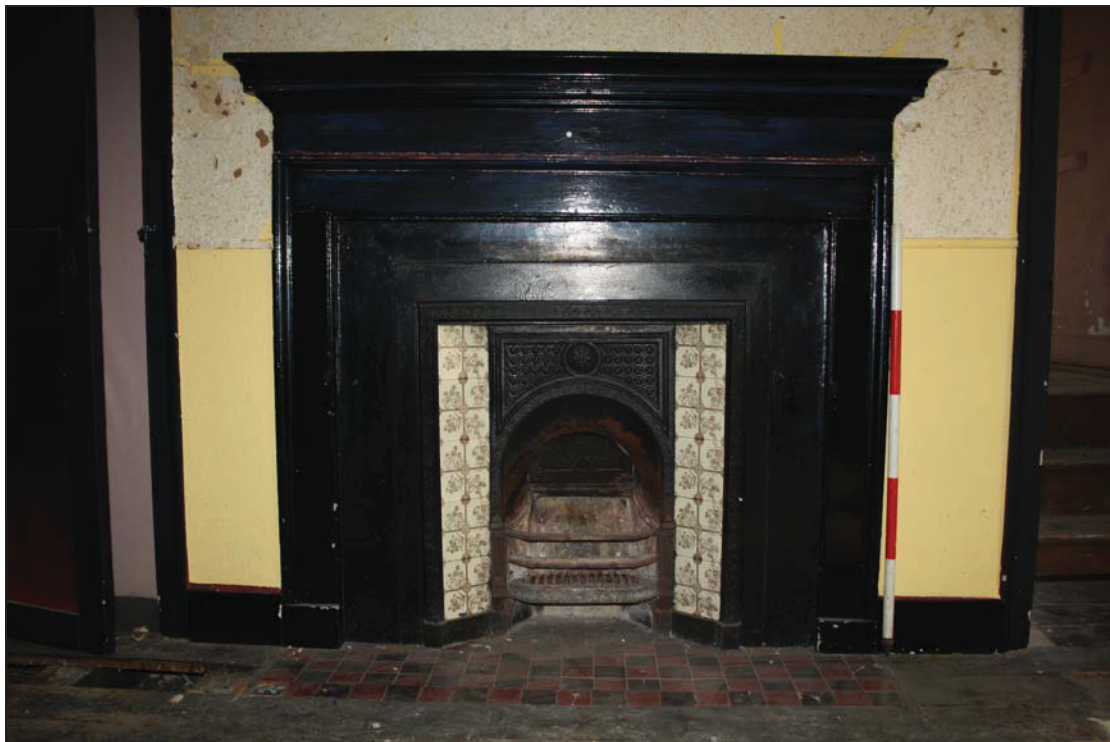
Plate 17 Fireplace with 18th century timber surround with later Victorian inset and hearth, FF02, taken from the south (DP 112)
