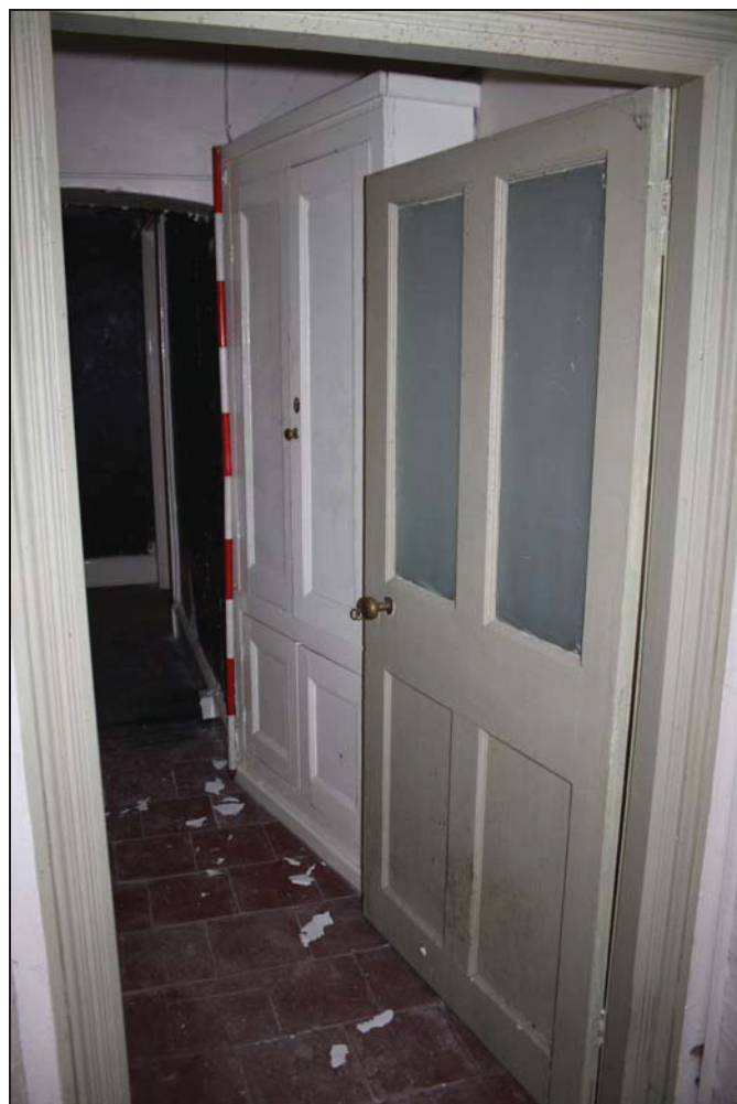
Plate 12 Cupboard, GF05, taken from the north (DP 34)
