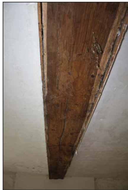
Hacked-back ceiling joist previously boxed in, FF03, taken from the east
