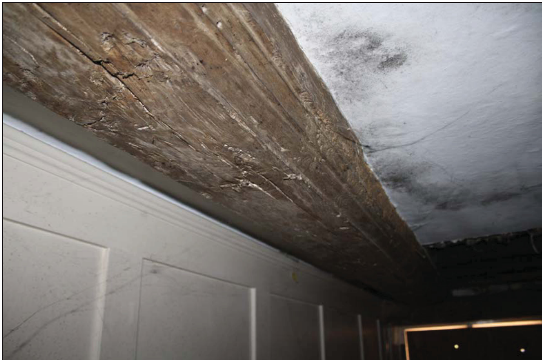
Plate 10 Moulded ceiling joist, GF03a, taken from the north-east (DP 55)
