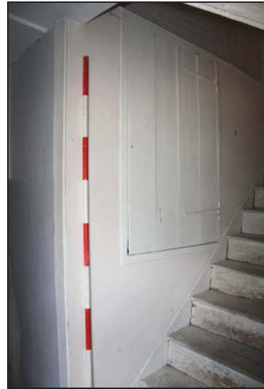
62 Cupboard located on the service range stair, taken from the south-east
