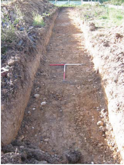
DP 13. Trench 6, looking south.
