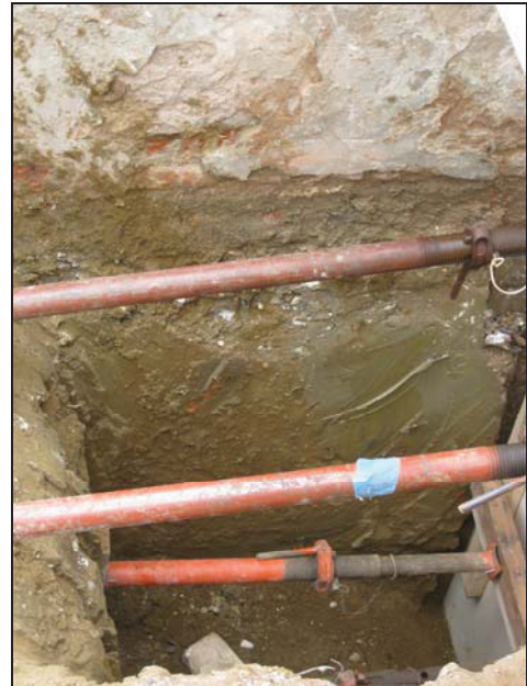
2 Sample Section 2. Looking west
