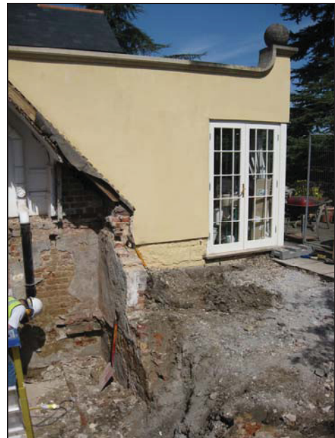
4 General view of the site. Looking north-east.
