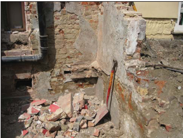
3 Existing cellar to be reduced. Looking north
