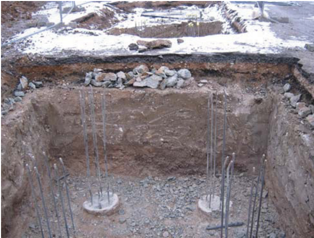
DP 19. S foundation trench. View N.
