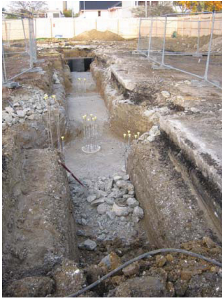
DP 13. E/central foundation trench. View N.
