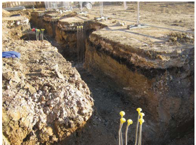
DP 6. W foundation trench. View NNE.
