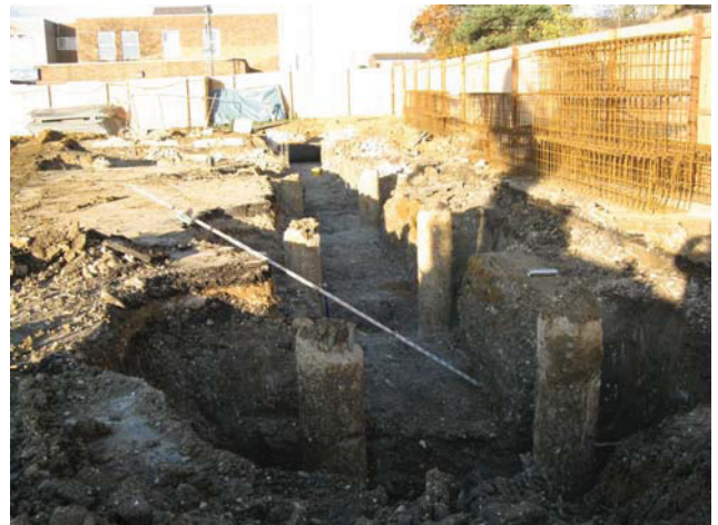
DP 16. E foundation trench. View NNE.
