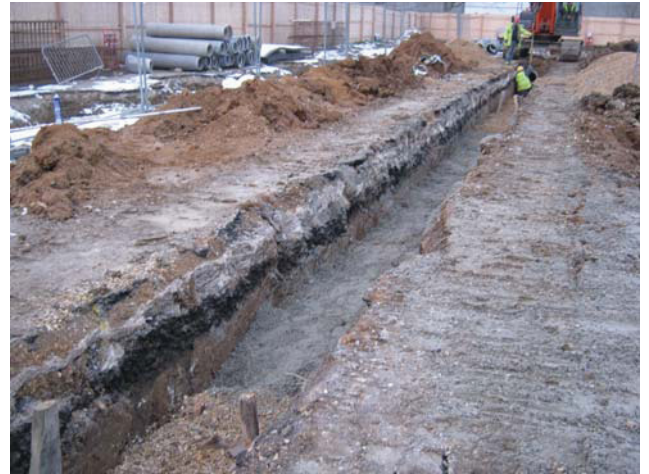
DP 20. Drainage trench in W part of the site. View NNW.
