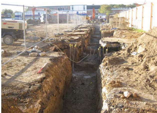
DP 5. W foundation trench. View S.
