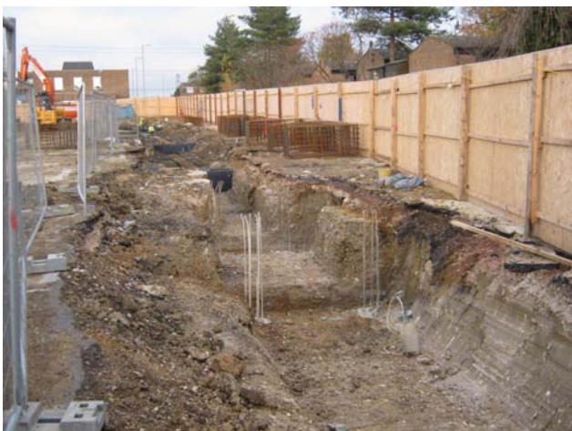
DP 17. E foundation trench. View NNE.
