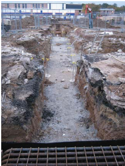
DP 11. W/central foundation trench. View S.
