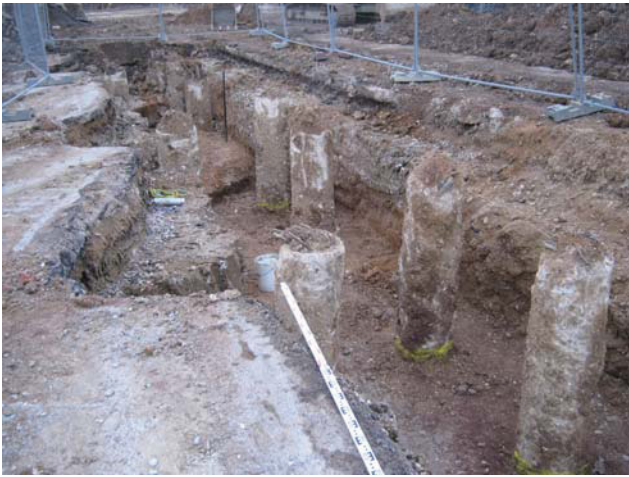
DP 9. W/central foundation trench. View SSW.
