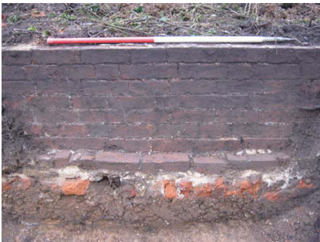
DP 5. Wall M1007. View NE.
