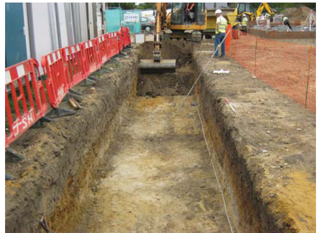
22 General view of soakaway 3 excavation. Looking east north-east.
