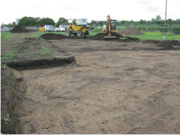
1 General view of the site during initial ground reduction. Looking west..
