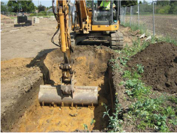
13 General view of soakaway 1 excavation. Looking north-east.
