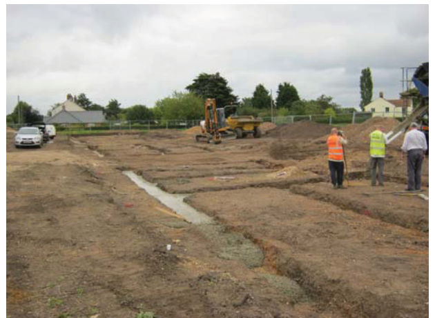
12 General view of footings nearing completion. Looking east.
