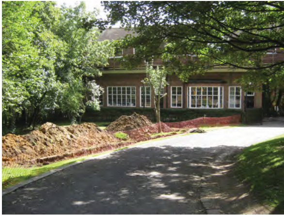
DP 1. The site during trenching works. View SE
