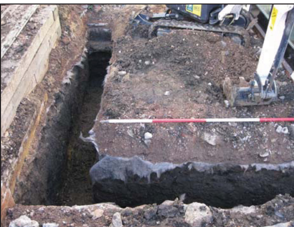
5 General photo. Looking NNW.
