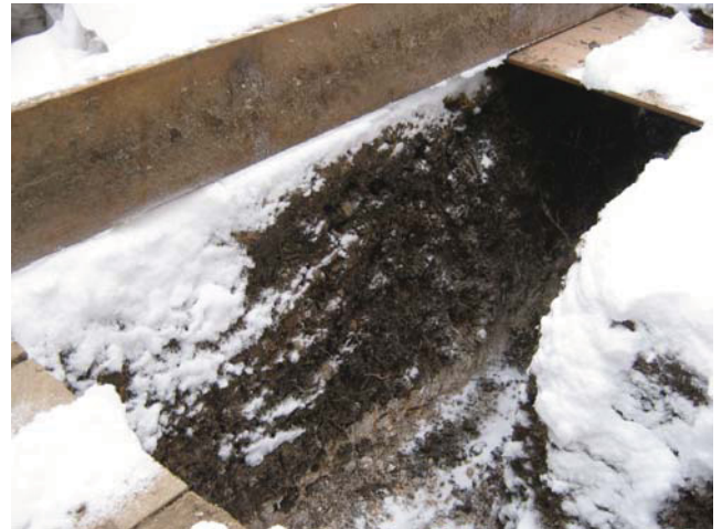
DP 4. N part of foundation trench. View ENE.
