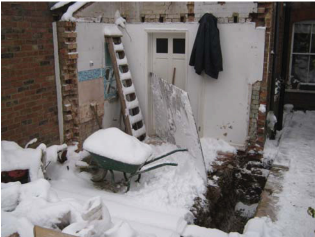
DP 3. The area of new extension. View SSW.
