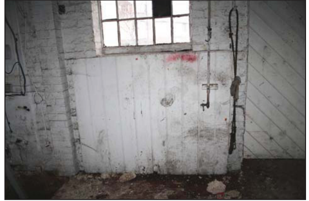
62 Section of match-lined boarding on the north wall of the main range (Building 1), taken from the south
