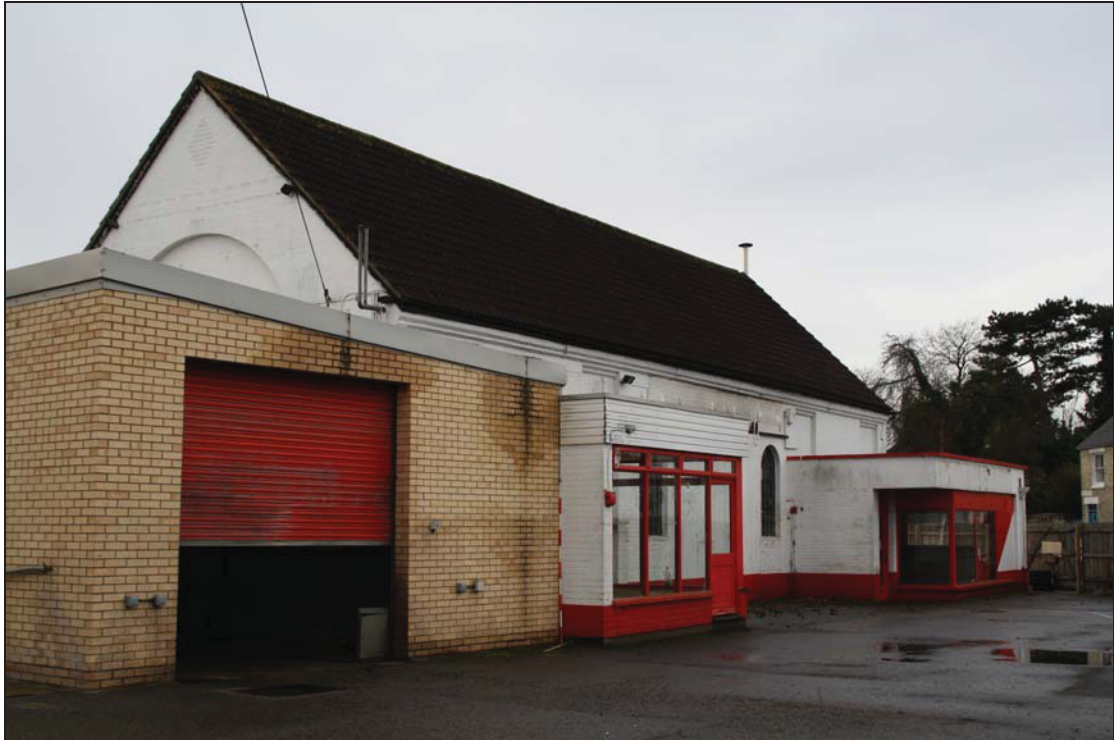
1 North side of Building 1 showing later additions, taken from the north-east (16)
