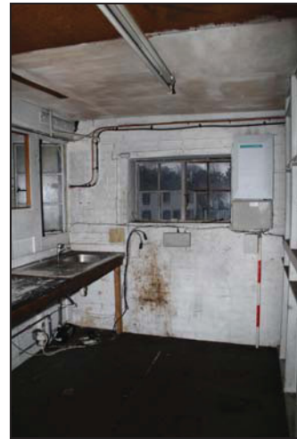
52 Enclosed room in the north-west corner of the mezzanine (Building 1), taken from the south
