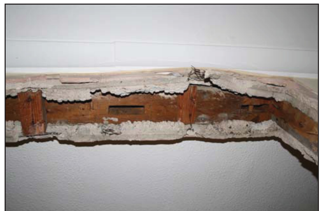
76 West wall of Room GF04 (Building 2) to the north showing exposed studwork covered with lath and plaster, taken from the north-east
