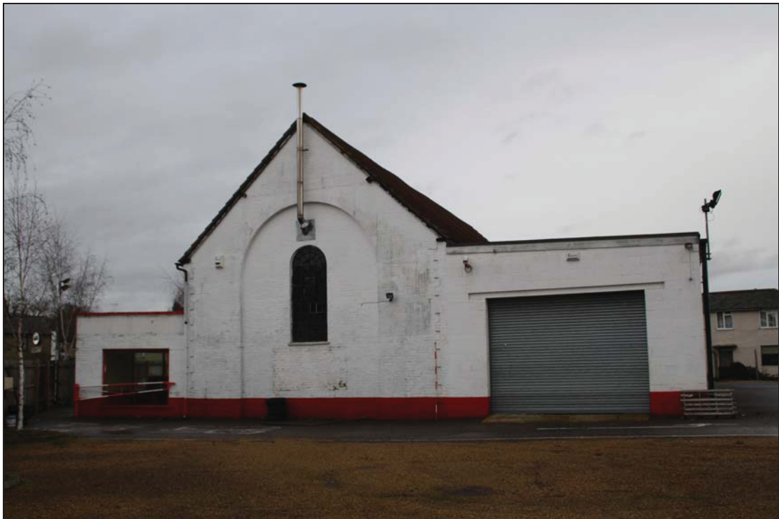
2 West elevation of Building 1, taken from the west (11)
