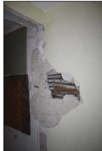
76 West wall of Room GF04 (Building 2) to the north showing exposed studwork covered with lath and plaster, taken from the north-east
