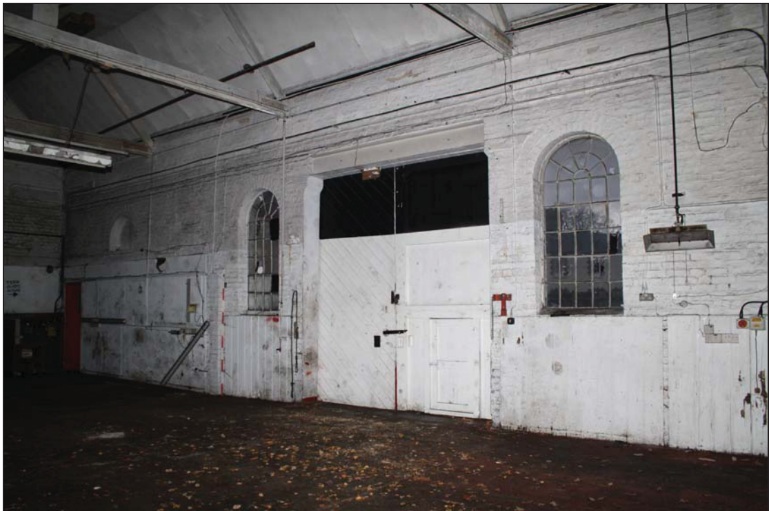
4 North wall of the main range (Building 1), taken from the south-east (41)
