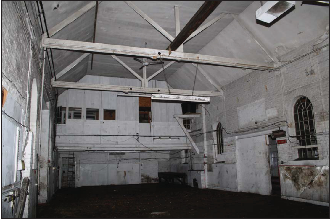
3 Interior of Building 1, taken from the west (36)
