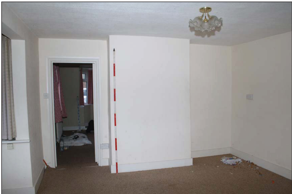
8 North side of Room GF02 (Building 2), taken from the south (24)
