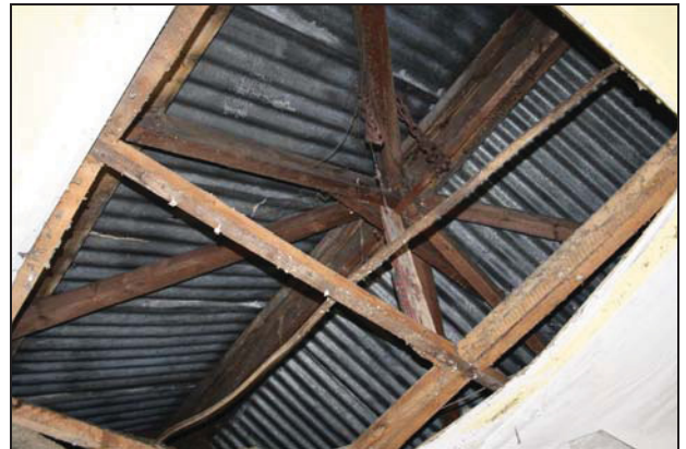
82 View of the roof structure of Building 3, taken from the west
