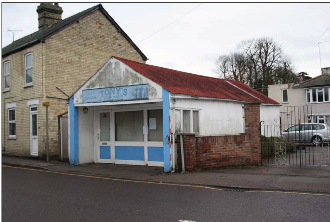
10 North and west elevations of Building 3, taken from the north-west (01)
