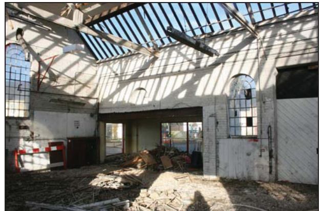
94 View of the east end of Building 1 after removal of the ceiling and exposure of the roof trusses, taken from the west
