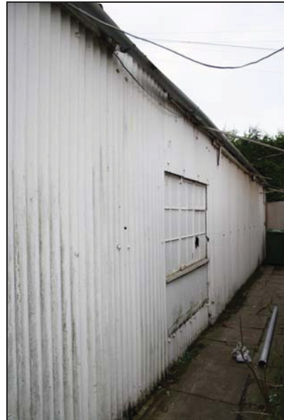
70 East wall of Building 3, taken from the south
