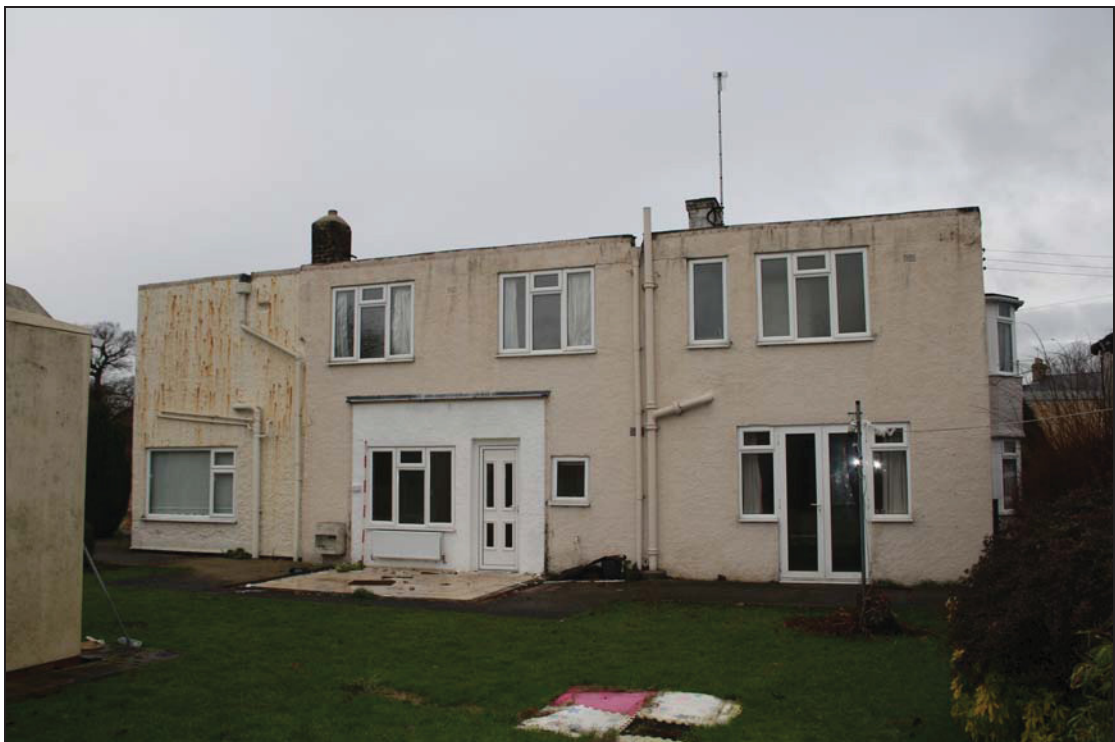
6 West elevation of Building 2, taken from the west (8)
