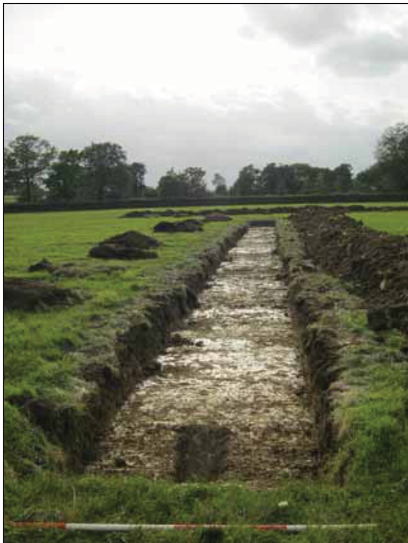
5 Trial Trench 5. Looking south-west
