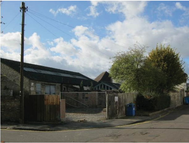
1 Site before evaluation, looking south-west
