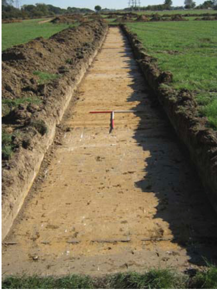
DP 43. Trench 262. Looking east.
