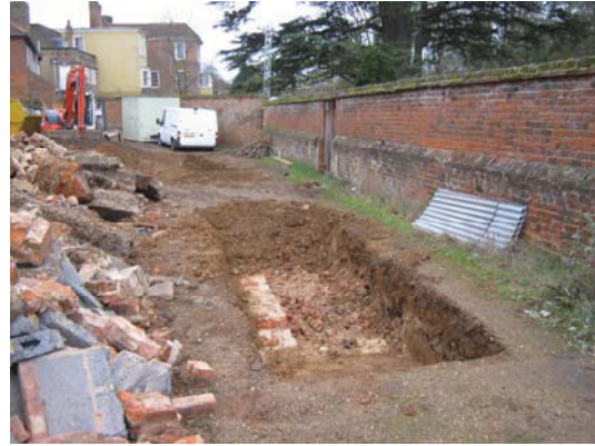
DP 2. Trench 2. Looking south.
