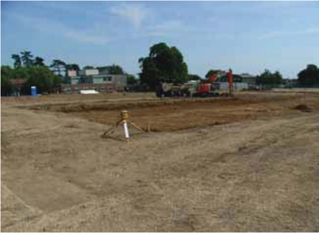
DP1. General photo of cut and fill operation, looking S.
