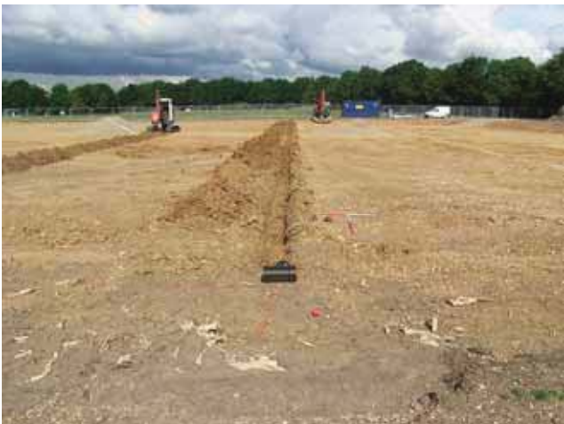
DP15. Lateral drains, looking NW.
