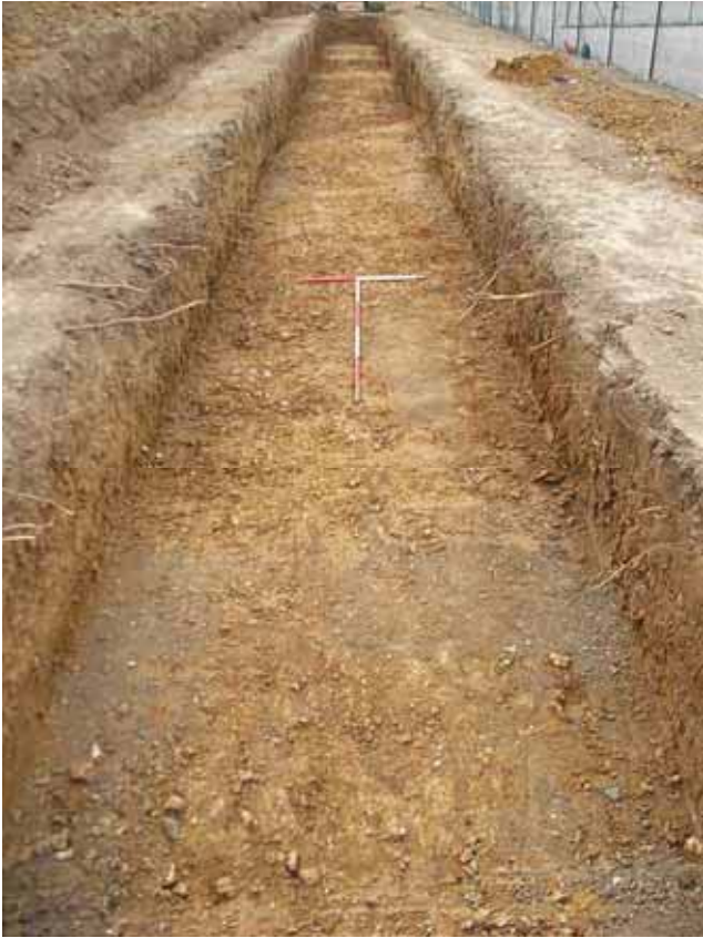
DP13. Soakaway trench post-excavation photo, looking SE.
