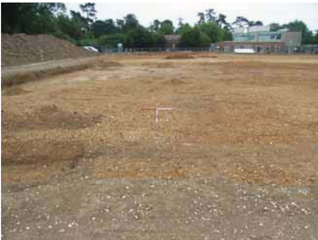
DP11. Pitch area post-excavation photo, looking SE
