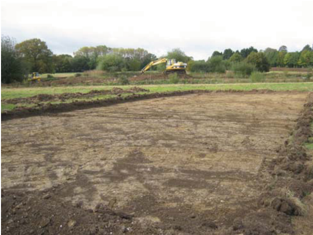
DP 3. Area 3. Looking south.
