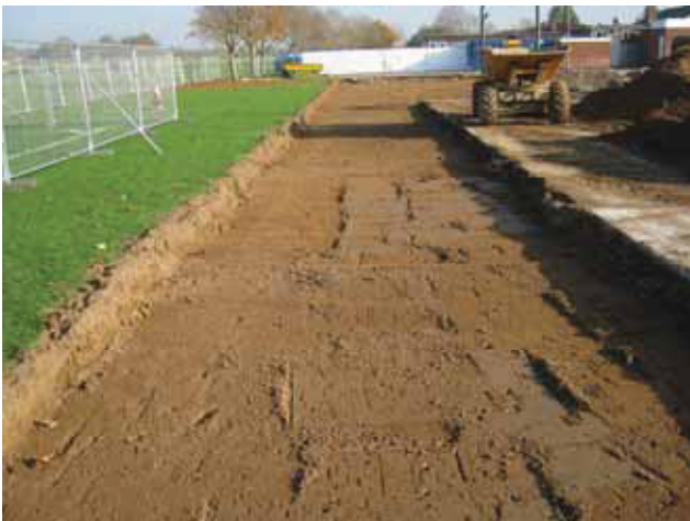
DP 3. Area of new car park. Looking east-north-east.
