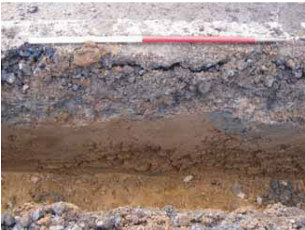
DP 15. Service trench. Sample section 5. Looking west-south-west.
