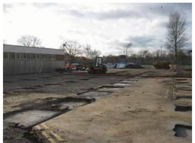
DP 12. Completed foundation pads. Looking south-west.
