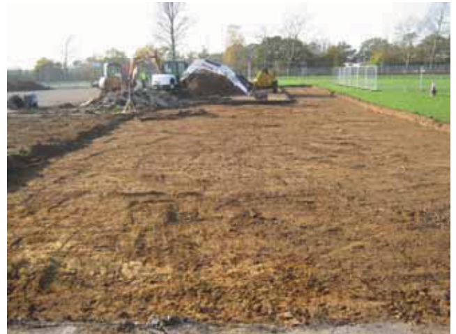
DP 2. Area of new car park. Looking west-south-west.
