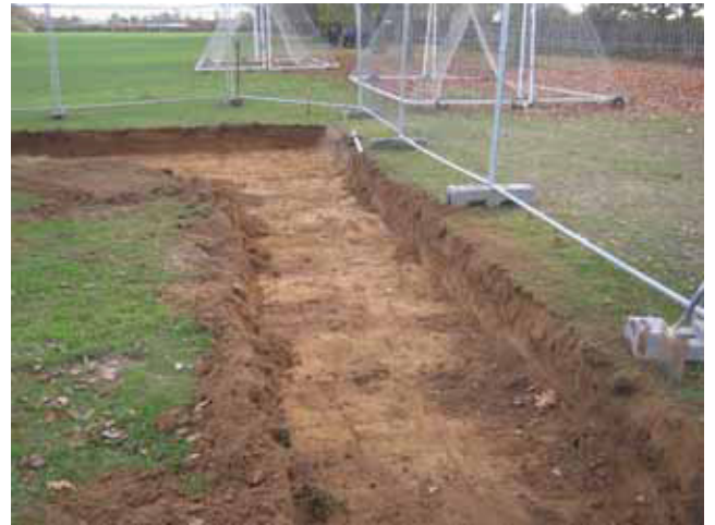
DP 8. Excavation of area of new cycle shelter. Looking south.
