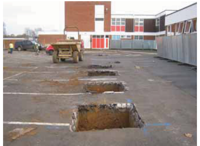
DP 10. Excavation of pits for foundation pads. Looking east-north-east.
