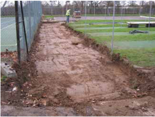
DP 7. New footpath to tennis practice area. Looking west.
