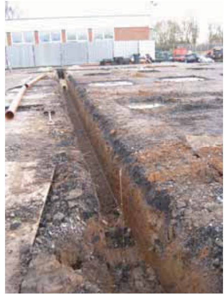
DP 14. Service trench. Looking south.
